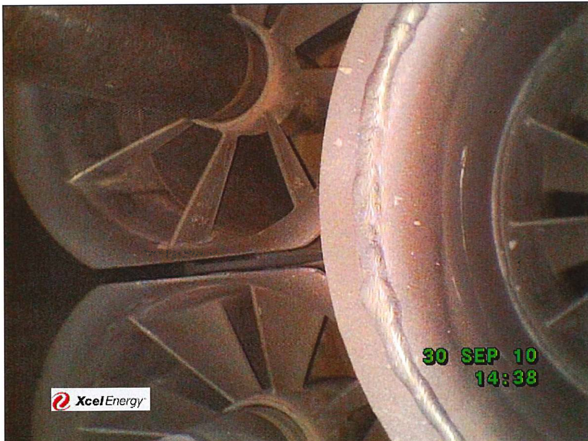
Main nozzle and rocket tip from the opposite side of #3 burner. Note how this rocket tip appears to be more centered in the guide tube. No obvious signs of any distress.
