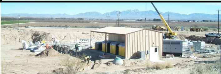
Doña Ana MDWCA WWTP Aeration Tanks and Clarifier Channel
