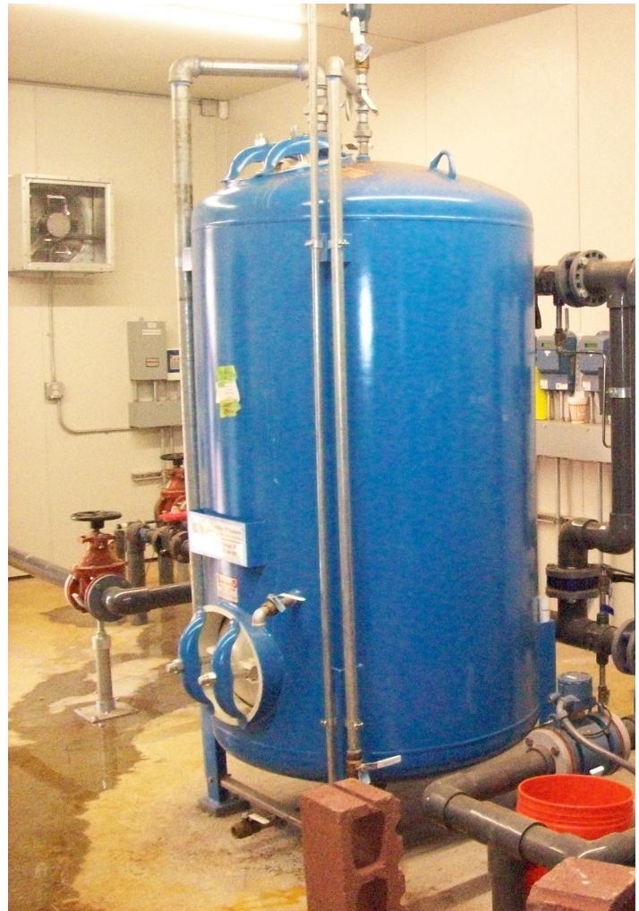
Algodones Arsenic Treatment System Funded by RIP and Capital Outlay
