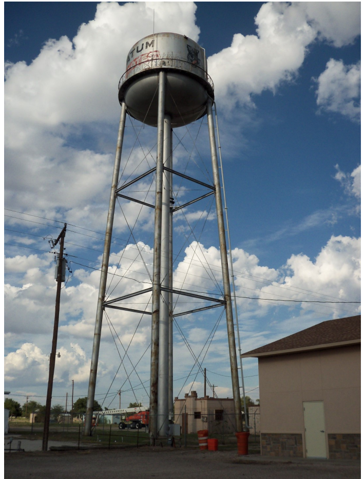
Tatum New Overflow Pipe for the Elevated Tank Funded by Capital Outlay
