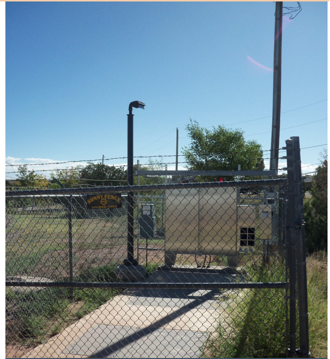
Santa Rosa Rehabilitated Pump Station Funded by CWSRF
