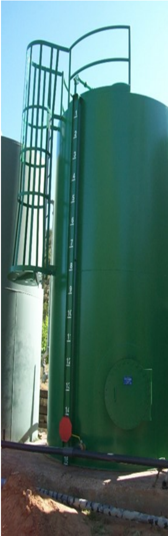
Placitas Water Storage Tank Funded by Capital Outlay
