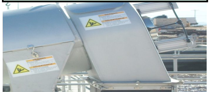
Doña Ana MDWCA WWTP Sludge Dewatering Screw Filter Press
