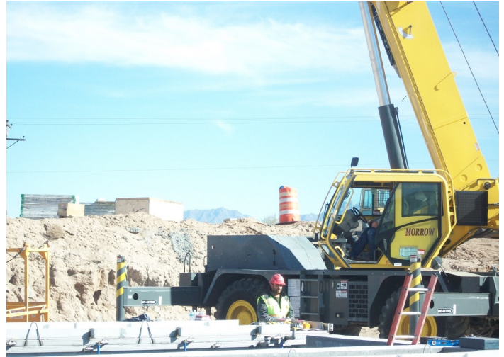
Doña Ana MDWCA WWTP Construction Funded by RIP
