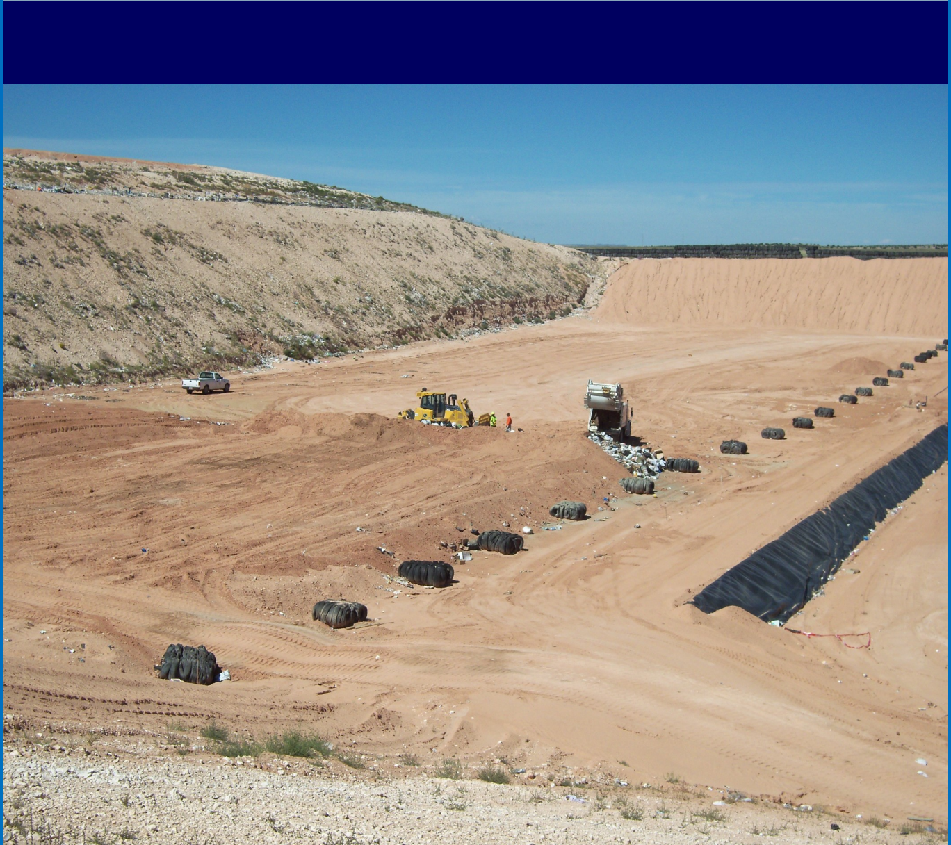
Estancia Valley Regional Landfill Cell Four Funded by CWSRF
