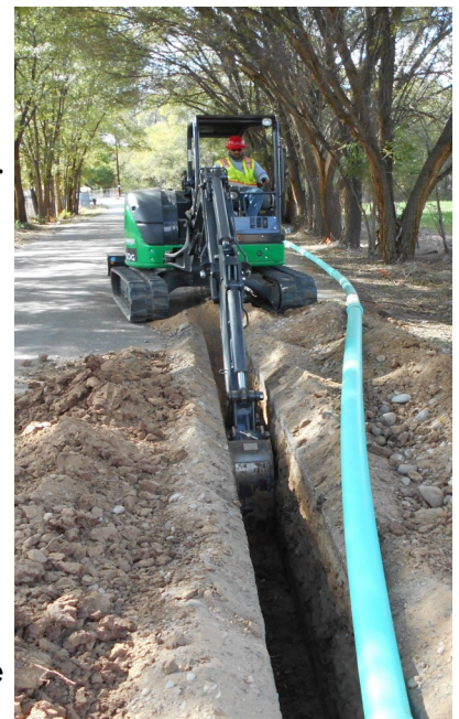
Town of Peralta Sanitary Sewer Project Funded by CWSRF
