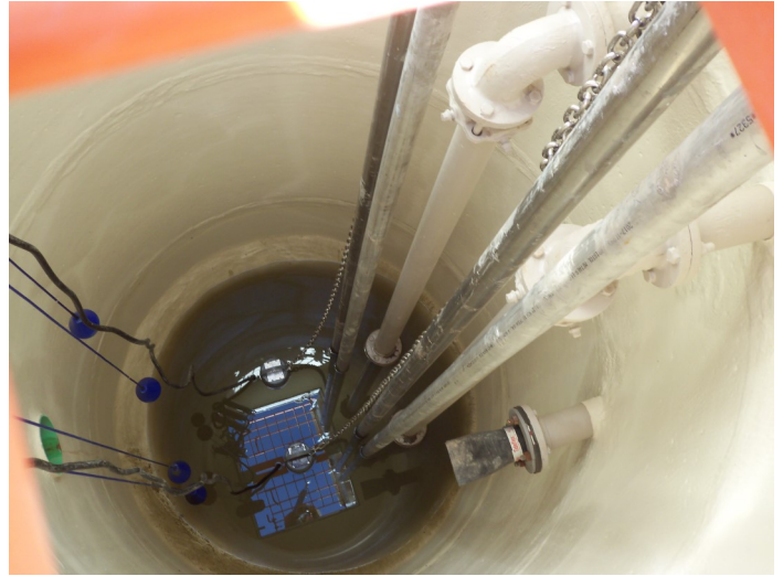
Edgewood Duplex Wastewater Pump Station Funded by Capital Outlay
