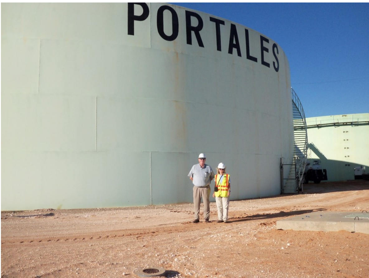
Portales Water Tank Replacement Project Funded by the Water Trust Board
