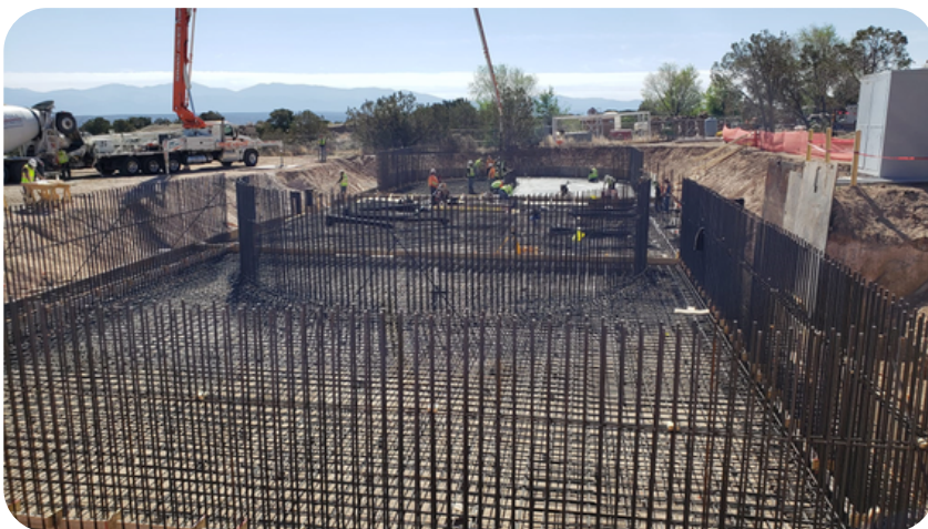
Construction of oxidation ditch and tertiary filter/ Ultra Violet disinfection building
