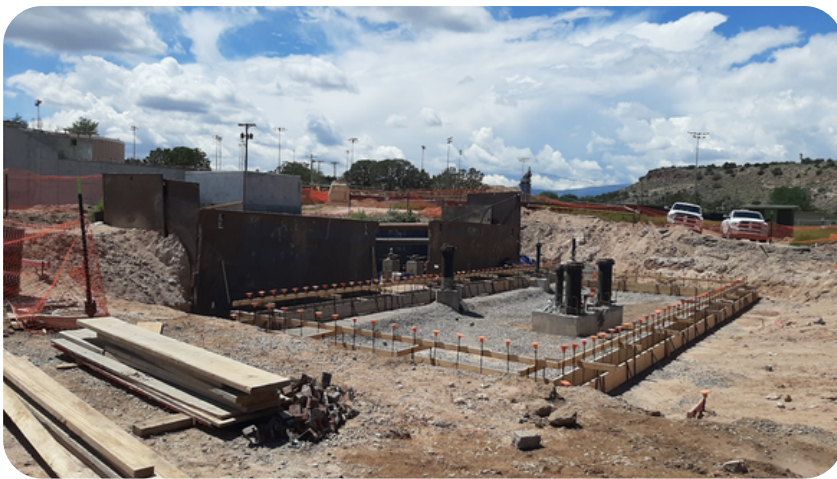
Construction of oxidation ditch and tertiary filter/ Ultra Violet disinfection building
