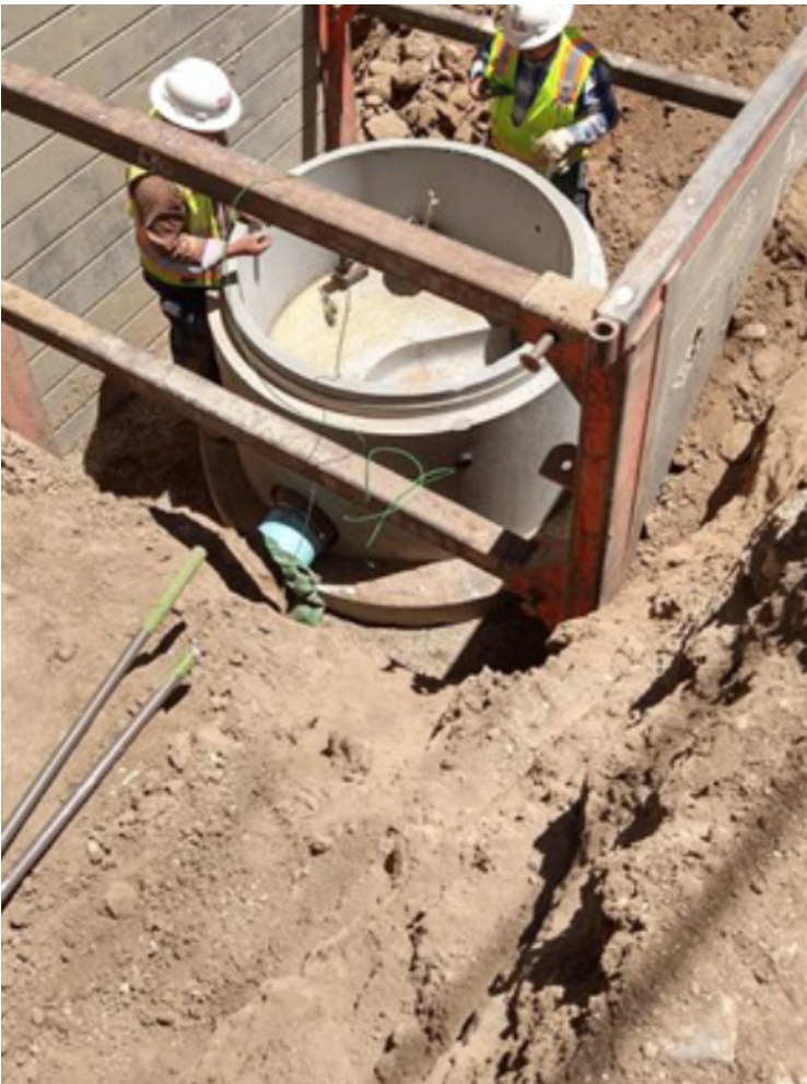
Manhole construction in the Village of Agua Fria
