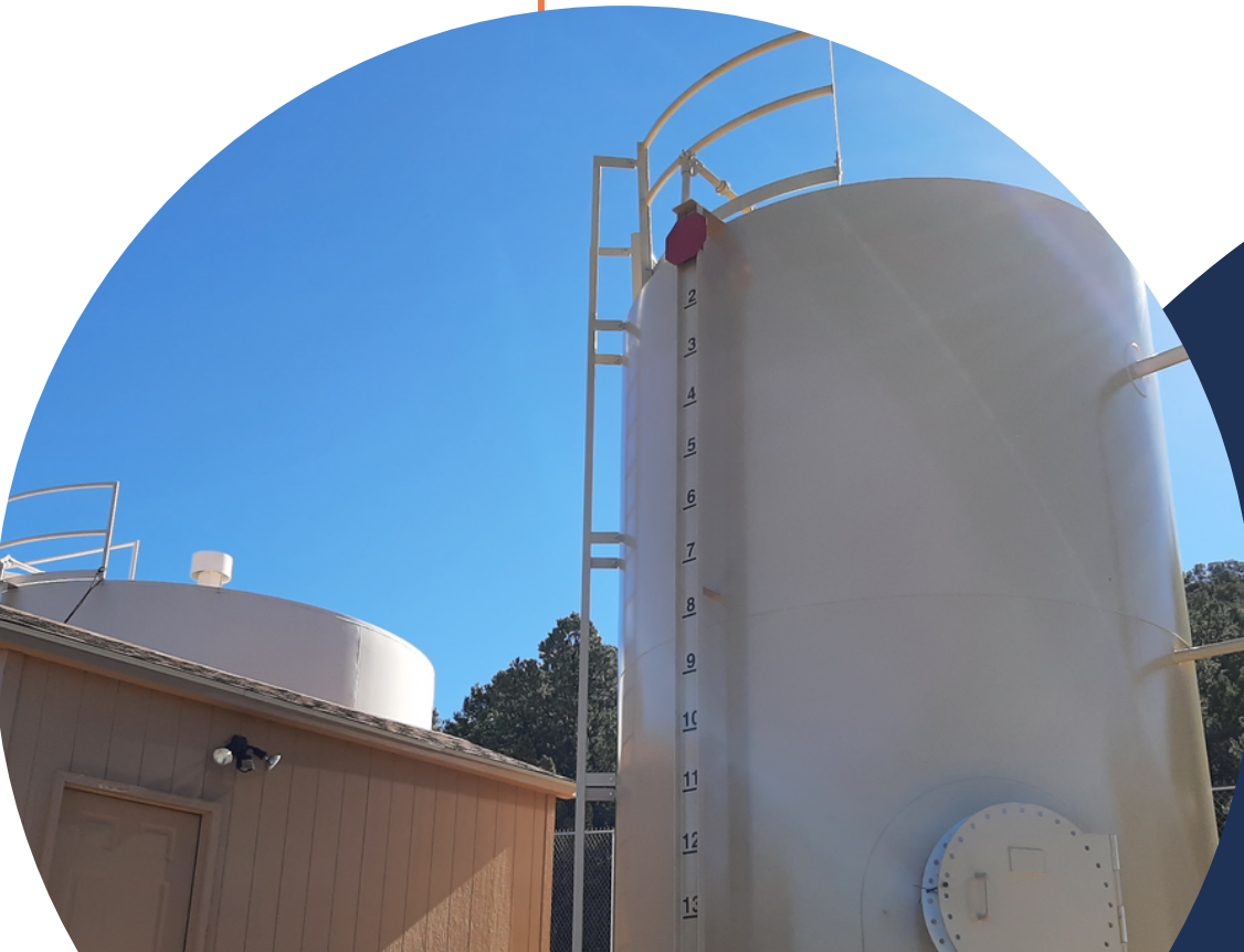
Upper Arroyo Hondo RIP 0035 Water Tank
