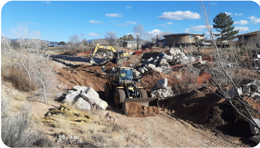
Construction of boulder retaining wall and boulder rundown channel
