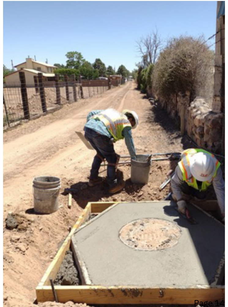
Manhole construction in the Village of Agua Fria
