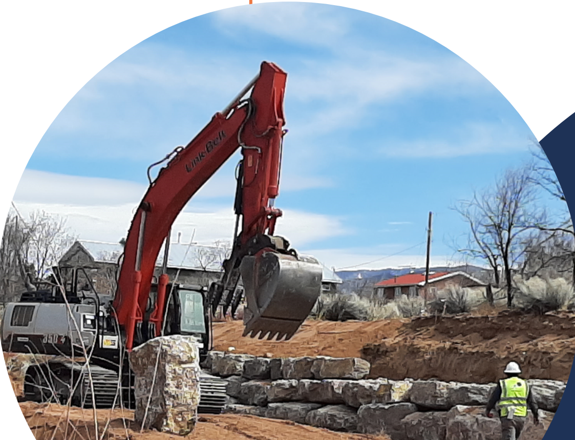
Santa Fe CWSRF 088 River Bank Stabilization
