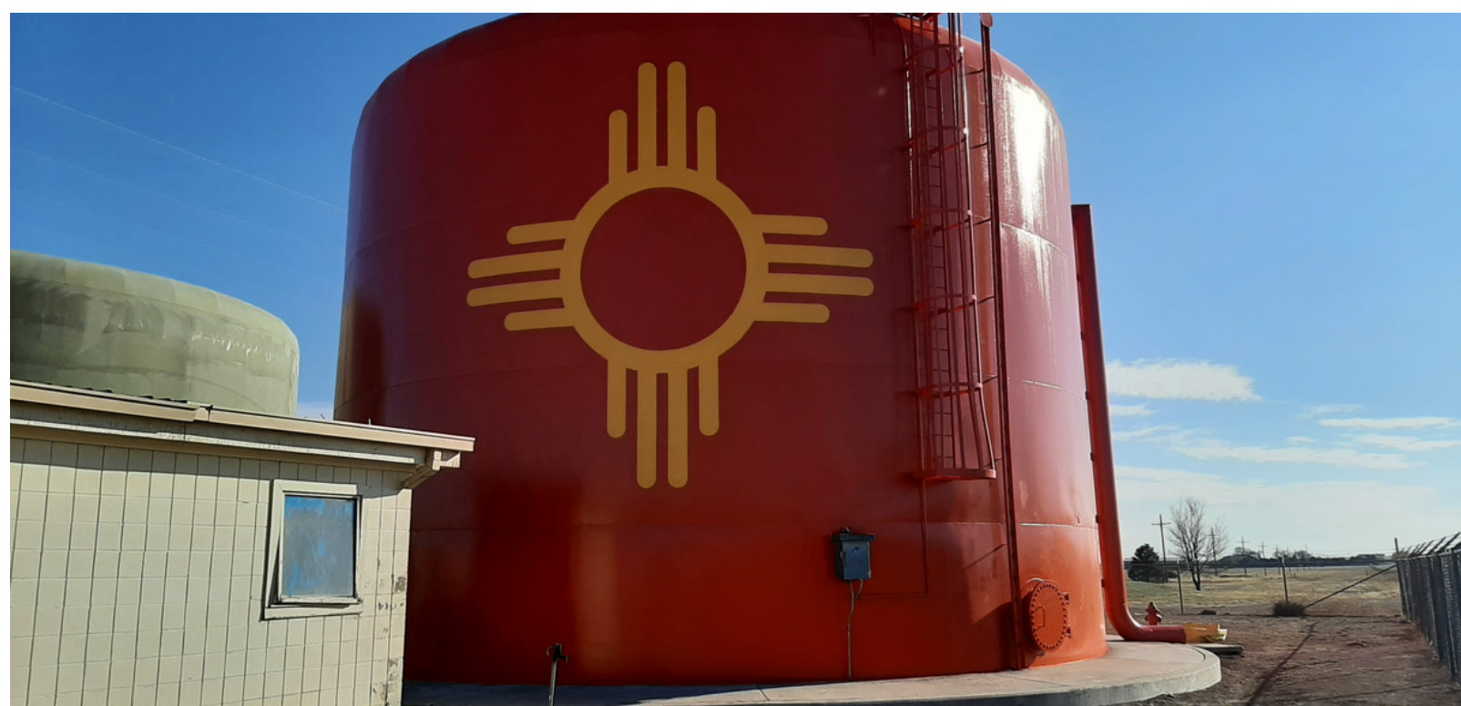
Clayton DW-5025 Tank Rehabilitation
