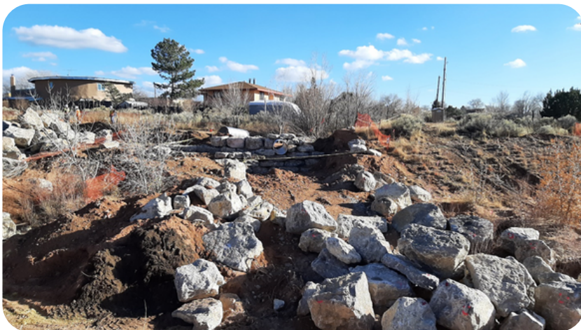
Construction of boulder retaining wall and boulder rundown channel
