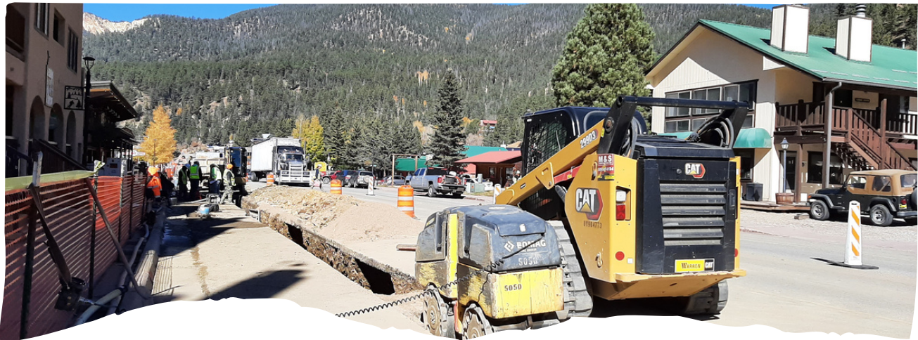
Town of Red River RIP 00038 Waterline Replacement.
