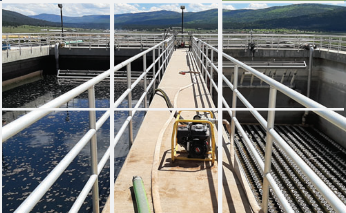
Village of Angel Fire CWSRF 107 Sequencing Batch Reactor Basins.
