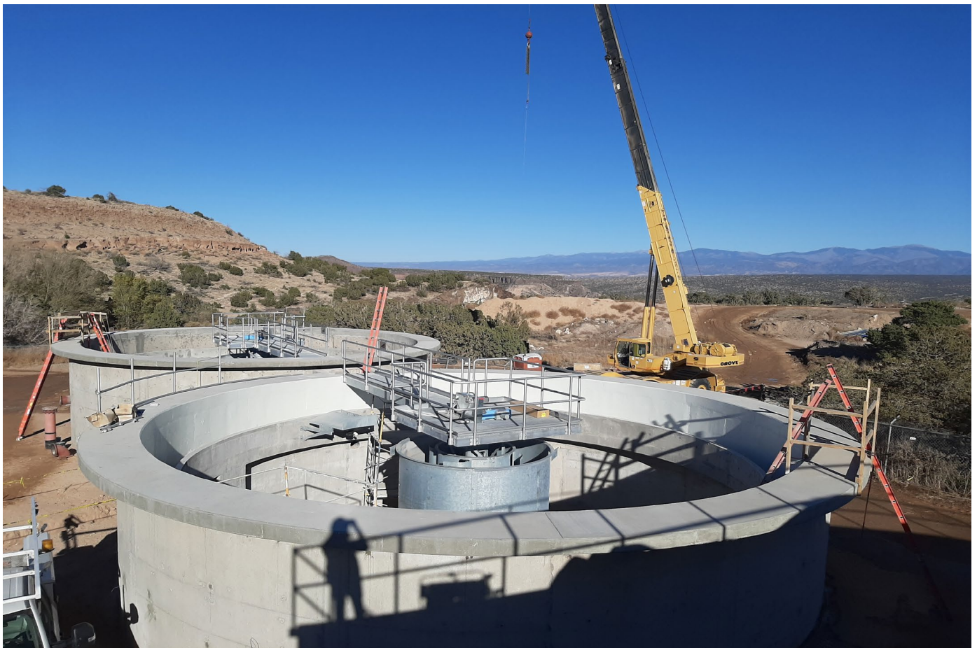
Los Alamos County White Rock Water Resource Recovery Facility Construction – CWSRF 110
