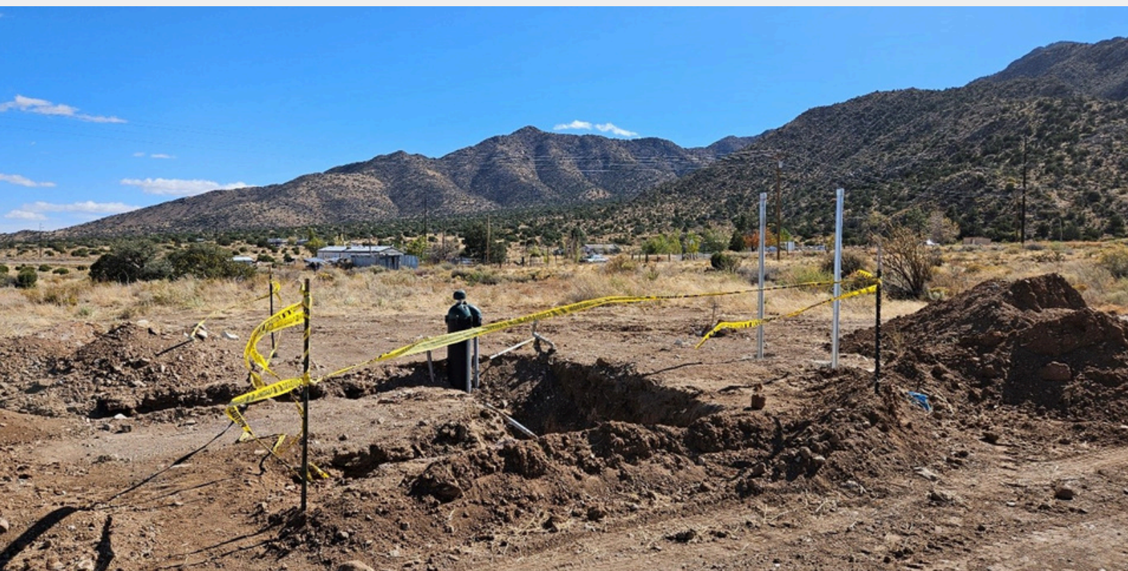
Village of Magdalena Trujillo Well Replacement Project: 5132-DW and 24-I2461-GF. Well Overview with Trenching for Electrical Services.
