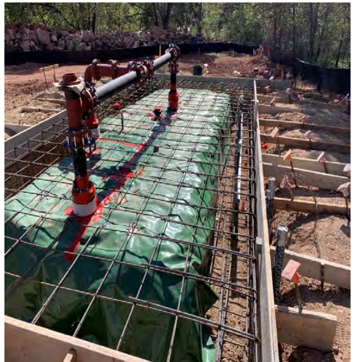
Tijeras Well No.3 Phase 2– Completed well house reinforcing bar installation
