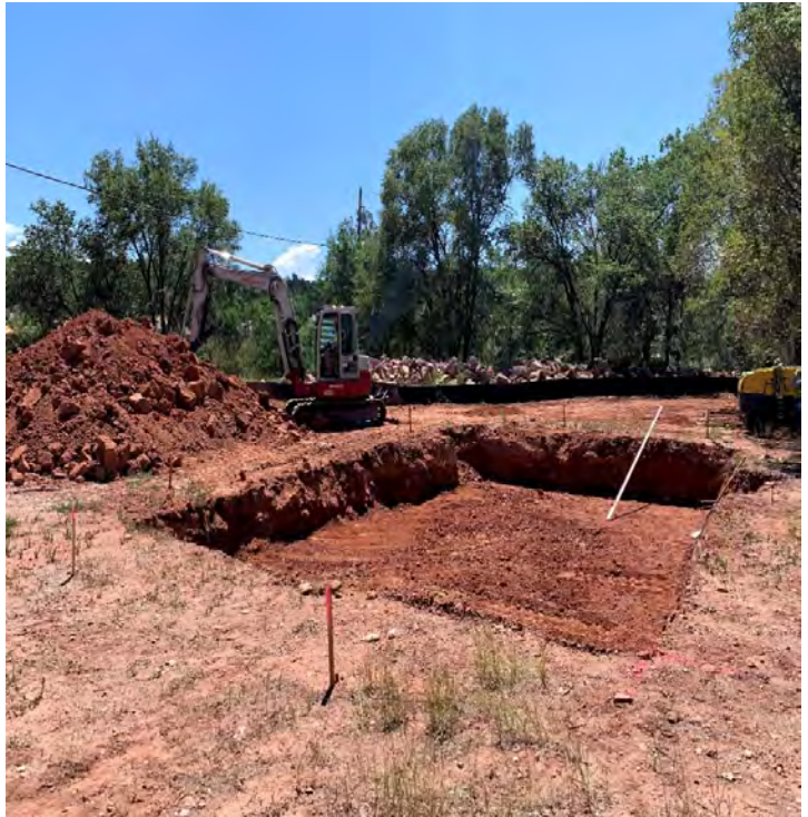
Tijeras Well No.3 Phase 2– Excavation for well house
