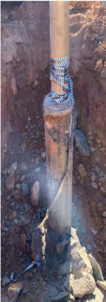
SAP 20-E2104-STB, Tijeras Well No. 3 Phase 2: Exposed well after excavation
