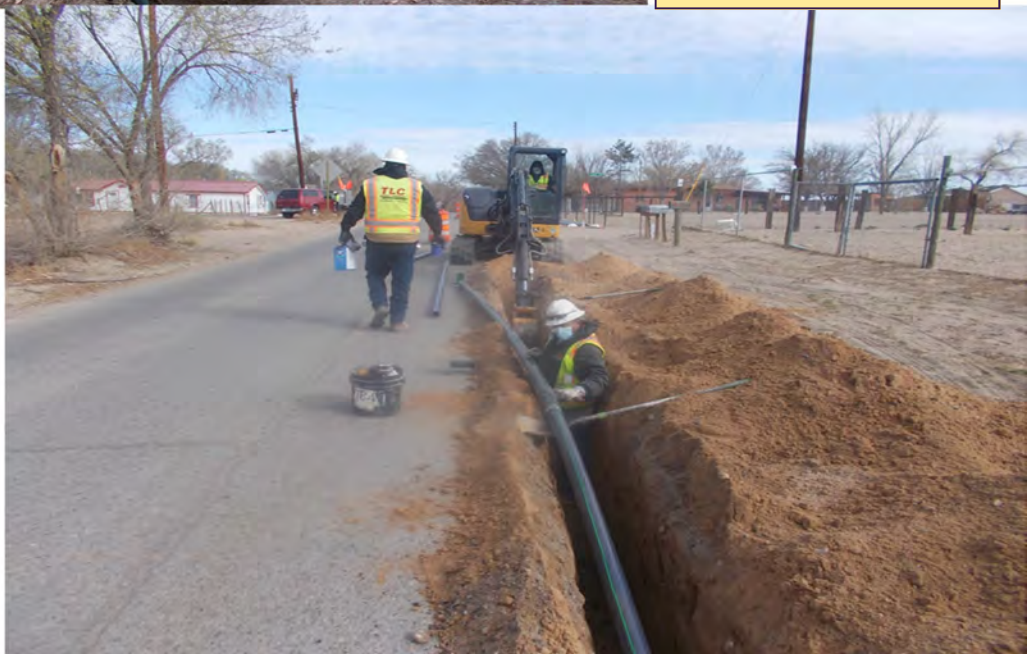
Construction of low pressure sewer collection line
