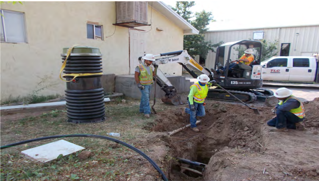
Construction of sewer service connection with grinder pump
