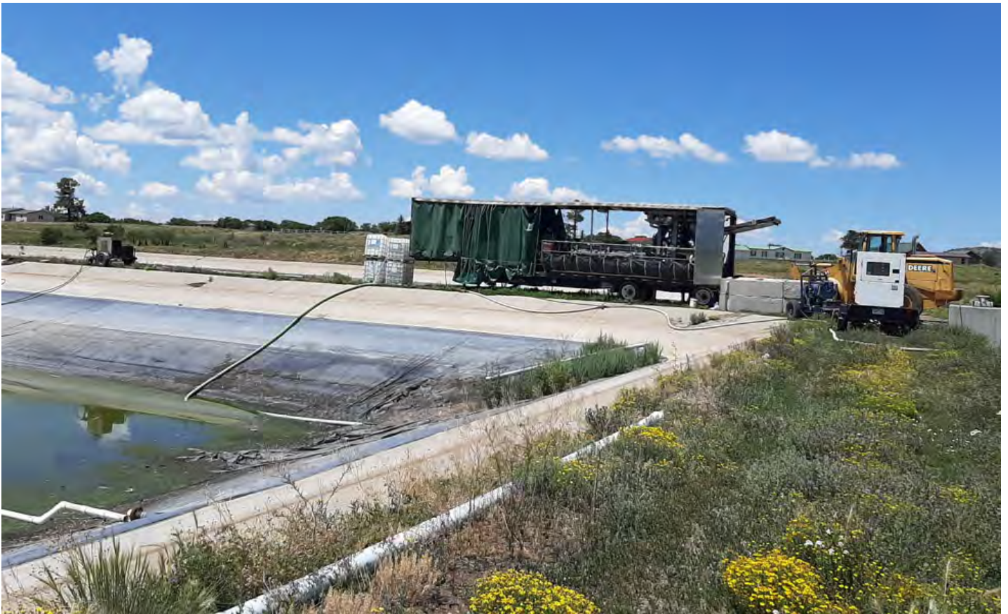
CWSRF Chama 066-Lagoon Decommissioning and Removal of Sludge
