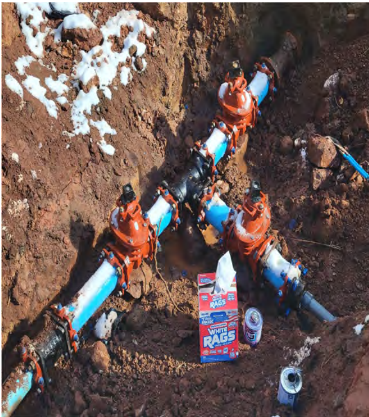
Brazos MDWCA Supplemental Well Development Connecting to Existing Water Main
