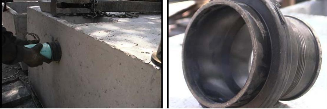
Figure 7. Neoprene collar seal with clamp
