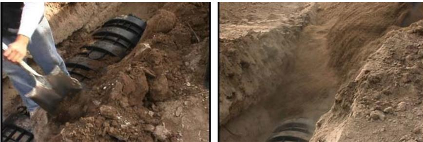
Figure 18. Once the chambers are placed backfill the sides of the chamber prior to backfilling the trench. Failure to do this may result the chambers collapsing.
