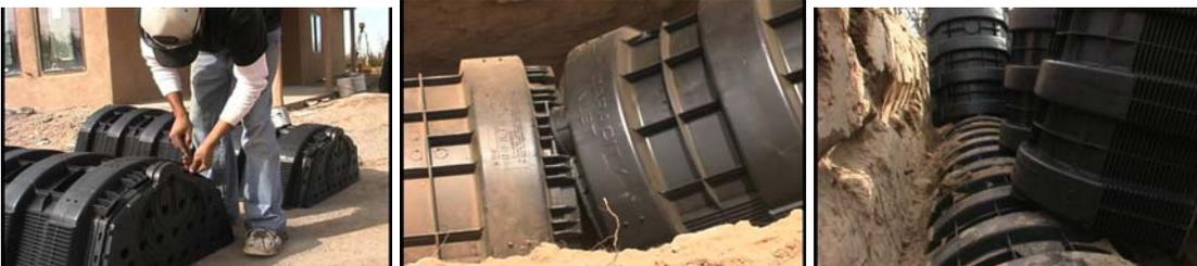
Figure 17. Screw in the end plate and then place the chambers in the trench in sequence.
