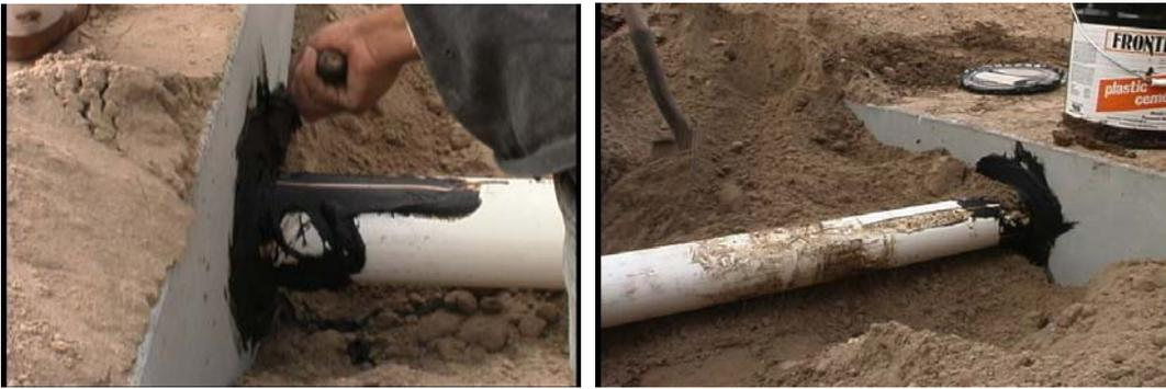
Figure 8. Pipe inlet/outlet joint showing seal
