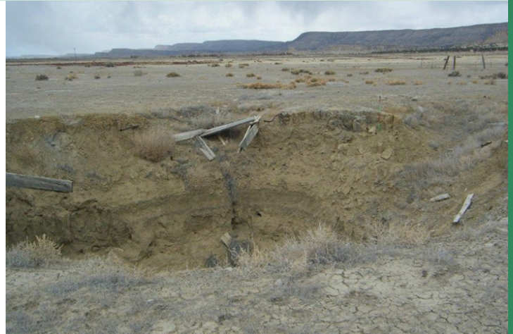
A large sink hole at a neglected AUM site in New Mexico. Neglected AUM sites may pose a physical danger to New Mexicans from pits, shafts (vertical entrances), adits (horizontal entrances), exposed waste rock, and other unstable mine structures.
