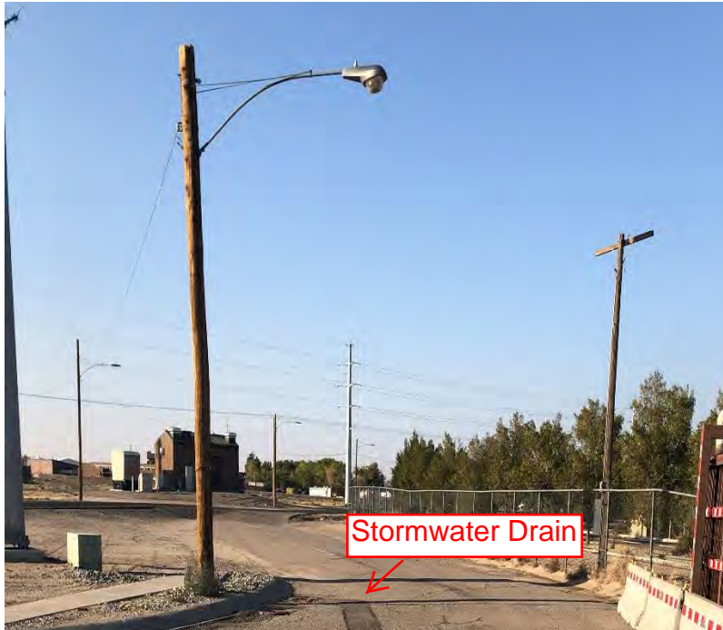
Location: Looking South at stormwater drain. Date: 10/6/2020
