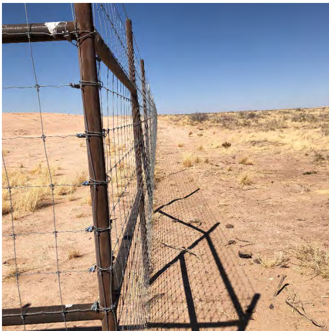
Figure 22SP-1 – View north from southeast corner of Catalina Recycling Containment #1. 32 32 49.34, -104 19 30.21
