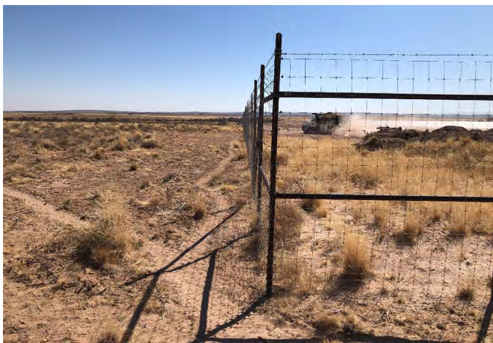
Figure 22SP-2 View south from northeast corner of Catalina Containment #1
