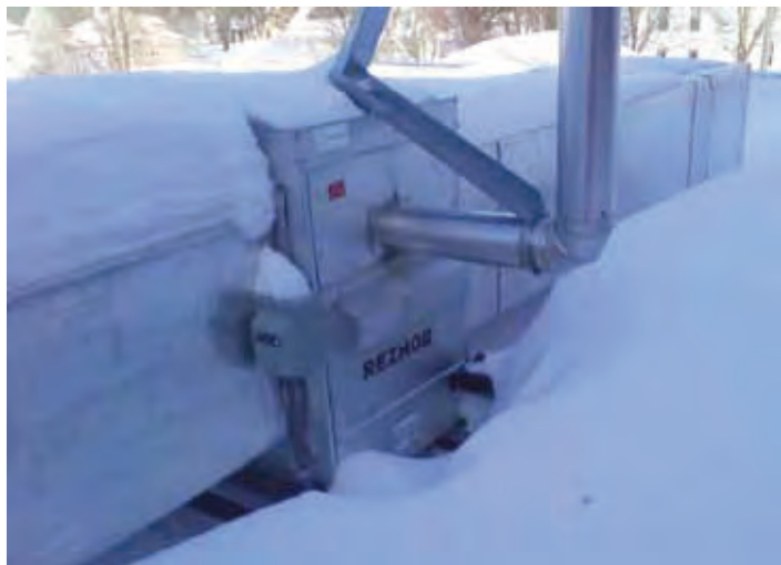
Reznor Rooftop Mounted Duct Furnace
