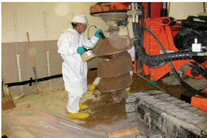
11. Auger Soil Removal and Field Screening
