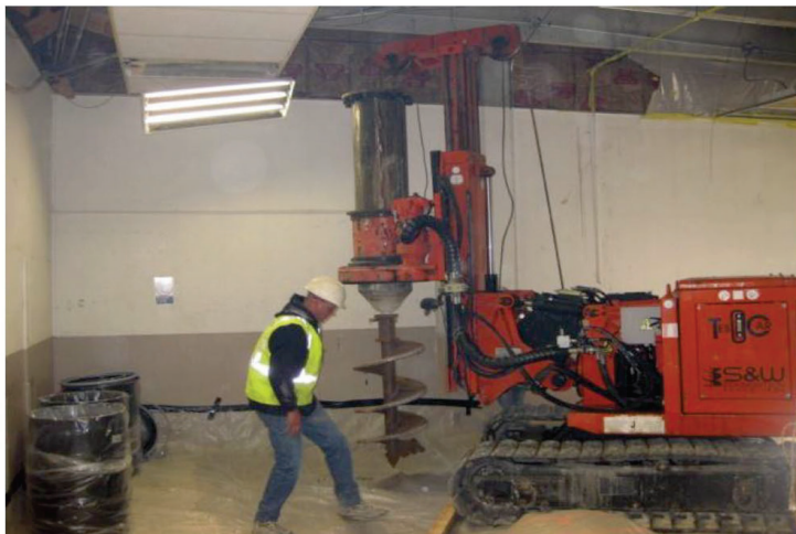
10. Bucket Auger Rig Set-up for Deep Soil Column Removal
