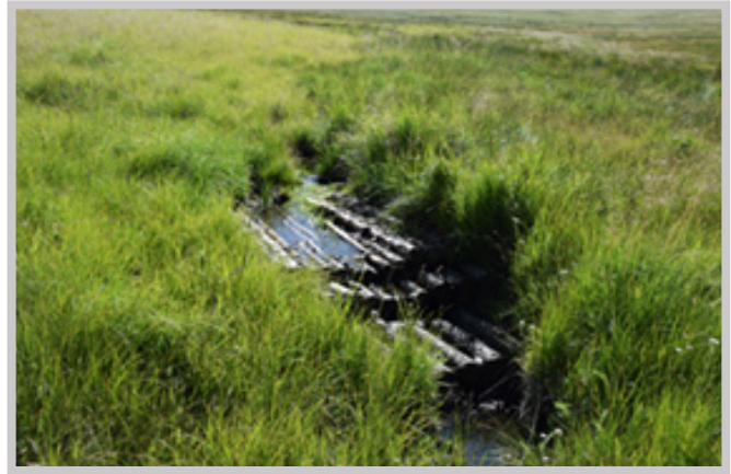
Grassy Creek. Log-rock rundown structure (left), and log step fall structure (right) in 2016, two years after installation.
