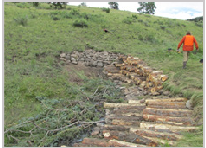
Springwagon Creek. A large headcut that was treated with a log stepfall structure. The photos were taken before and immediately after construction in 2016.
