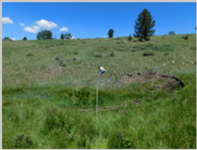
Springwagon Creek. A large headcut that was treated with a log stepfall structure. The photos were taken before and immediately after construction in 2016.
