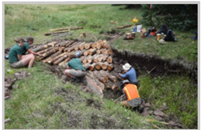
Grassy Creek (left) and Springwagon Creek (right). Volunteers building log step fall structures to arrest erosion in headcuts, preventing the slope wetlands upstream from drying. The crew boss of each crew is wearing an orange vest.
