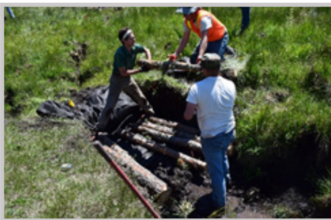
Grassy Creek (left) and Springwagon Creek (right). Volunteers building log step fall structures to arrest erosion in headcuts, preventing the slope wetlands upstream from drying. The crew boss of each crew is wearing an orange vest.
