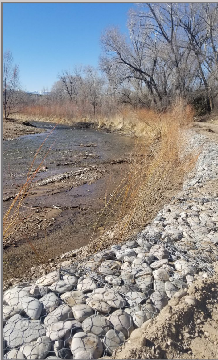
Rio Embudo, looking upstream near Dixon, February 20, 2020 with newly planted willow stakes along the base of the gabion wall (left) and September 3, 2021 with fully established willows after two growing seasons (right).
