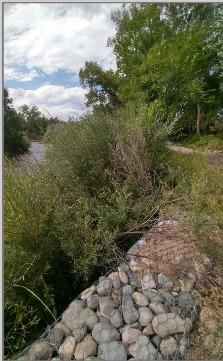
Rio Embudo, looking upstream near Dixon, February 20, 2020 with newly planted willow stakes along the base of the gabion wall (left) and September 3, 2021 with fully established willows after two growing seasons (right).
