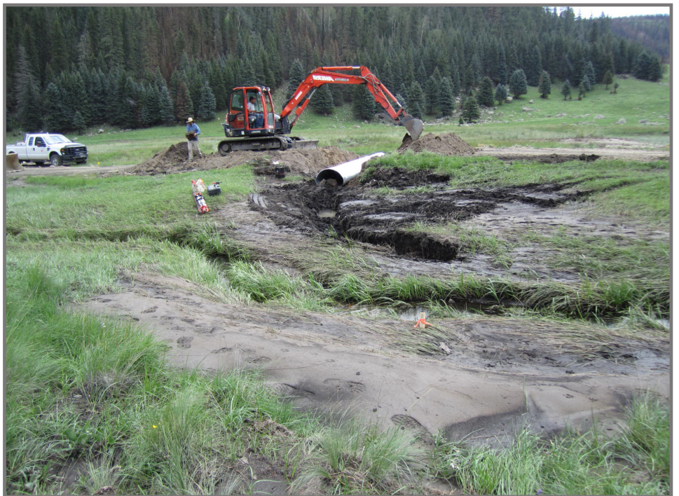
Improving the road crossing at the Rito de los Indios tributary confluence to reduce erosion.
