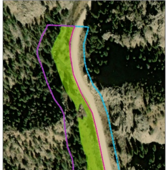
Figure 15. Roads can have direct and severe impacts on riverine wetlands, particularly in confined canyons where roads are commonly near the stream channel.
