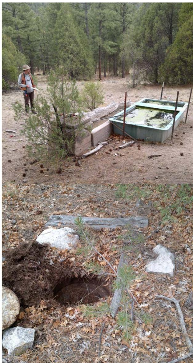
Fig. 3–27. All water is captured in tanks and springboxes at Harris Canyon Spring in the Gila National Forest.
