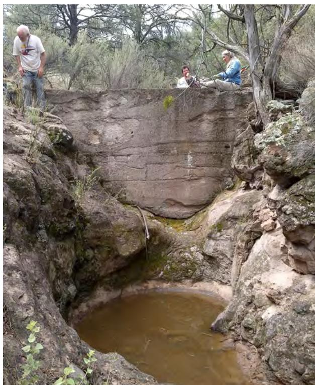
Fig. 8–8. Honey Bee Dam Spring in the Gila National Forest has been dammed, resulting in reduced natural physical disturbance. Also, the dam reservoir filled with sediment, eliminating its utility in flow regulation or impoundment.
