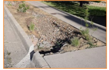
Silver City Harvesting stormwater to reduce sediment in San Vicente Creek
