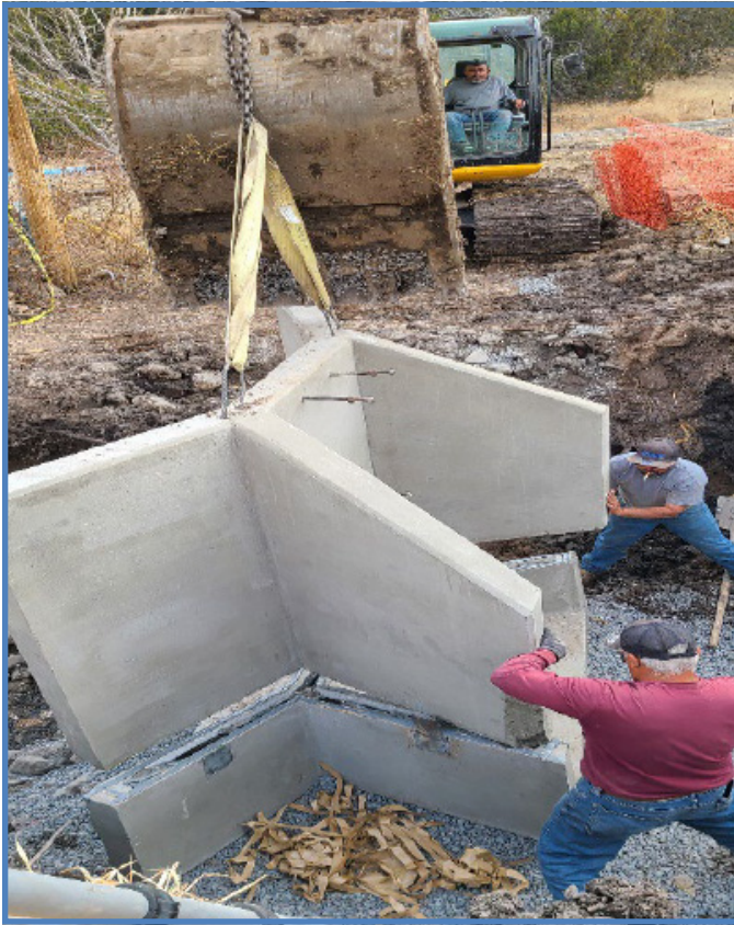
The RFO BLM constructing and installing a replacement headgate on the Government Spring Acequia near the Rio Bonito River in the Fort Stanton Snowy River Cave National Conservation Area (NCA).
