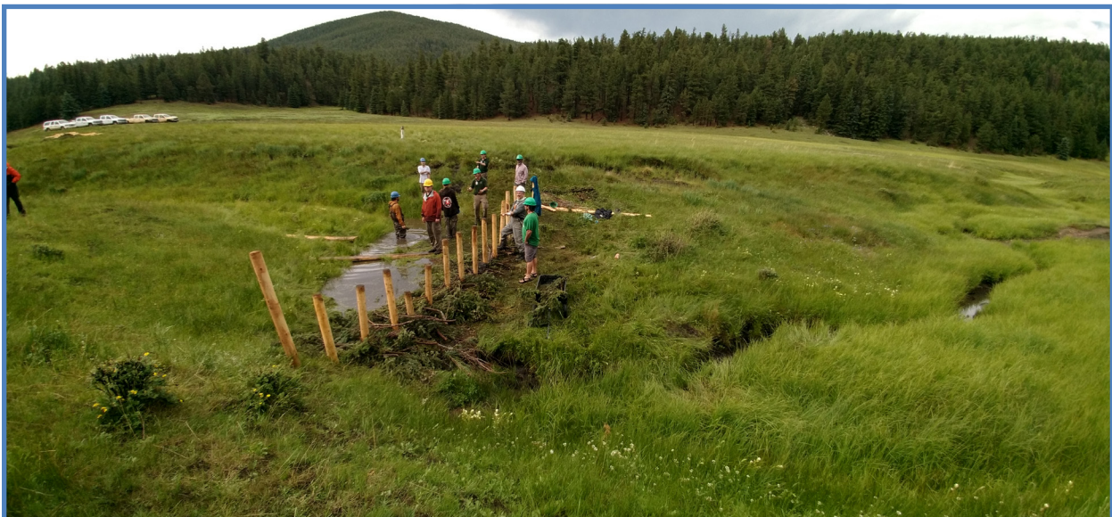
Beaver Dam Analog (BDA) built on the Philmont Boy Scout Ranch in northern NM during a workshop hosted by the Philmont Boy Scout Ranch and Anabranch Solutions.
