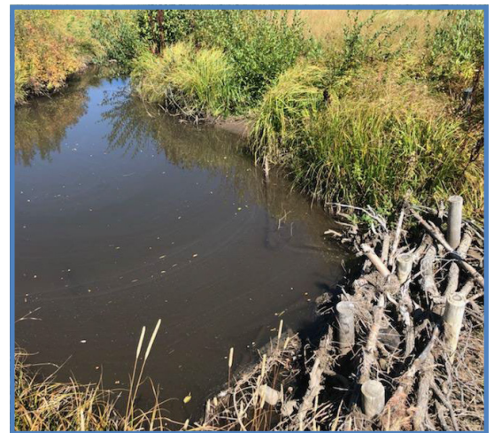
(Photo left) Natural recruitment of woody vegetation within an elk exclosure. (Photo right) Beaver Dam Analog maintenance.
