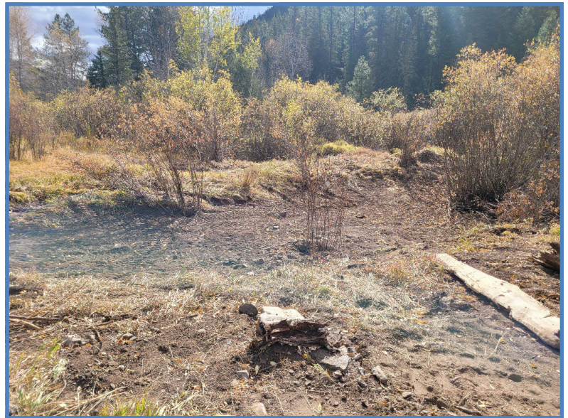
Dalton Canyon Water Quality Improvement Project – plug and pond/plug and spread treatment.
