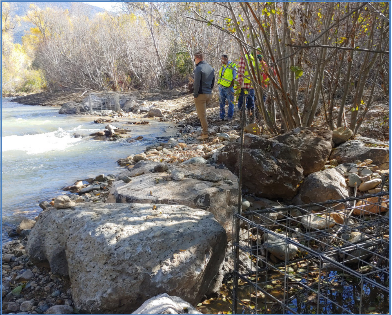
The Red River Aquatic Habitat Restoration Project. Pictured are two bank stabilization structures and two beaver pond levelers installed to prevent inundation of a nearby road.
