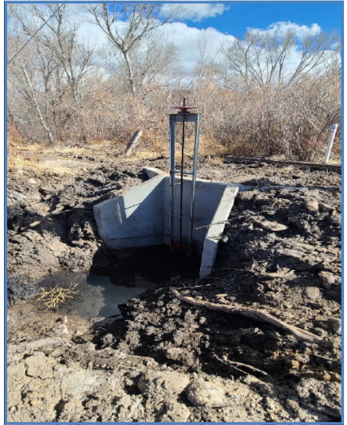
The RFO BLM constructing and installing a replacement headgate on the Government Spring Acequia near the Rio Bonito River in the Fort Stanton Snowy River Cave National Conservation Area (NCA).
