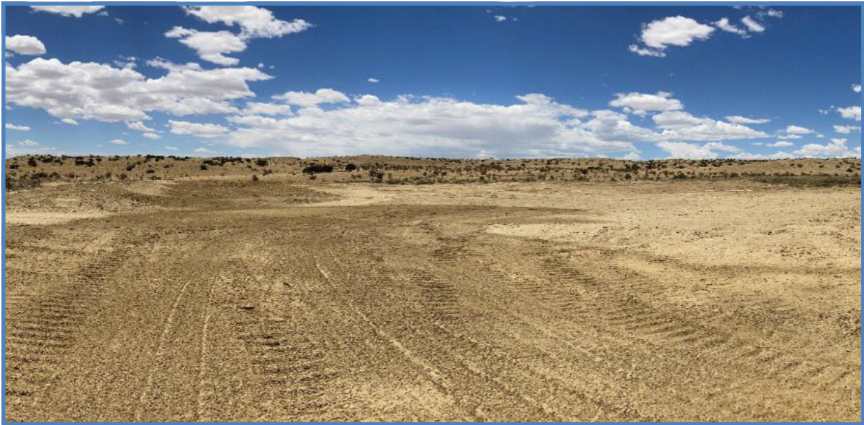
Panorama view of the Southwest Tank after removal of stored sediment (Photo courtesy of JJ. Gallegos)
