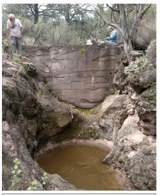
Fig. 3–31. Honey Bee Dam Spring in the Gila National Forest has been dammed, resulting in reduced natural physical disturbance. Also, the dam reservoir filled with sediment, eliminating its utility in flow regulation or impoundment.
