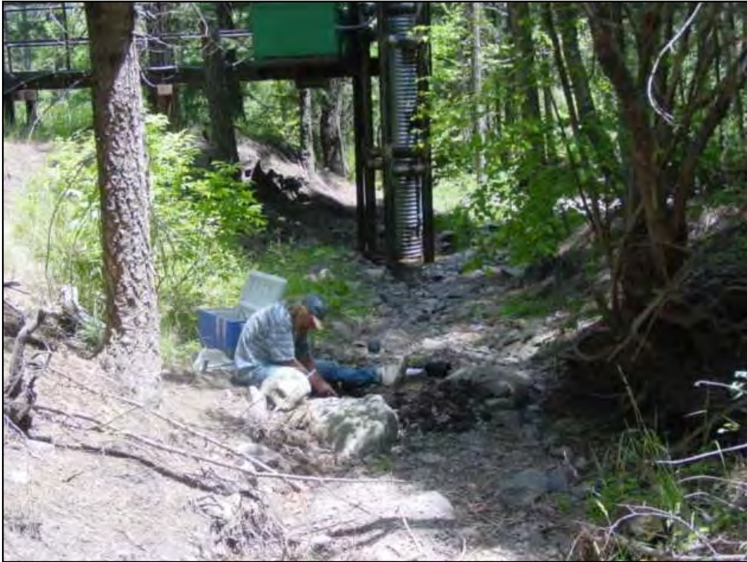
Installing Single-stage Sampler in Water Canyon, July 2006
