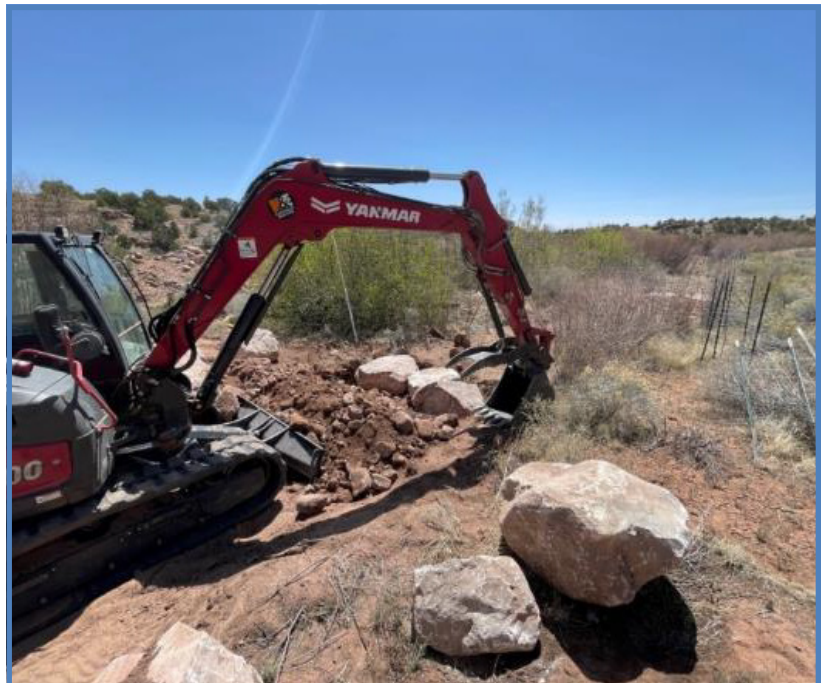
Photo right, One rock dam being built in Bluewater Creek.
