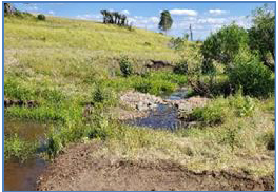
Constructed riffle in the Edward Sargent Wildlife Management Area.
