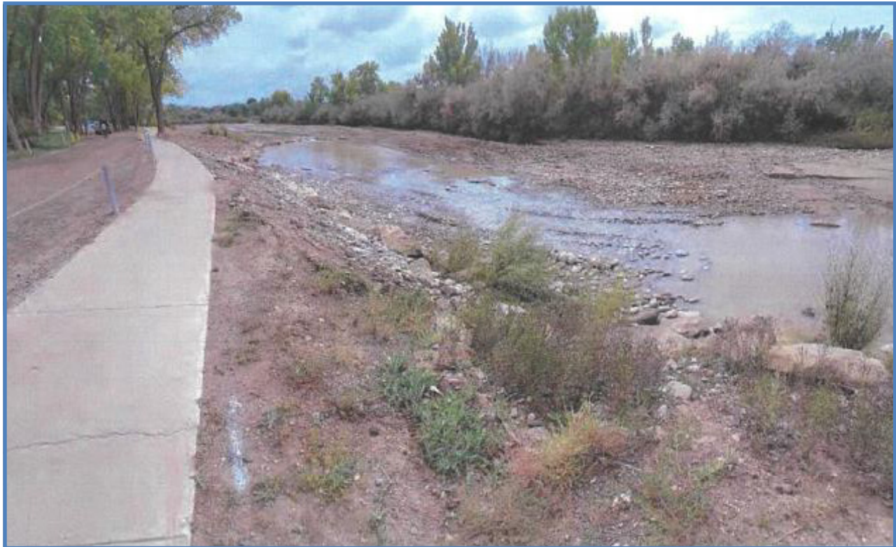
Photo above, Riverside Park, immediately following construction, looking upstream of the Animas River at the J-hook rock structure and pool in the distance for improved fish habitat and a bank step rock bench adjacent to the sidewalk in the foreground.
