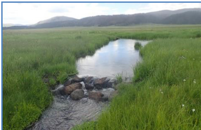
Photo above, One rock dam constructed just below a spring that feeds Jaramillo Creek.
