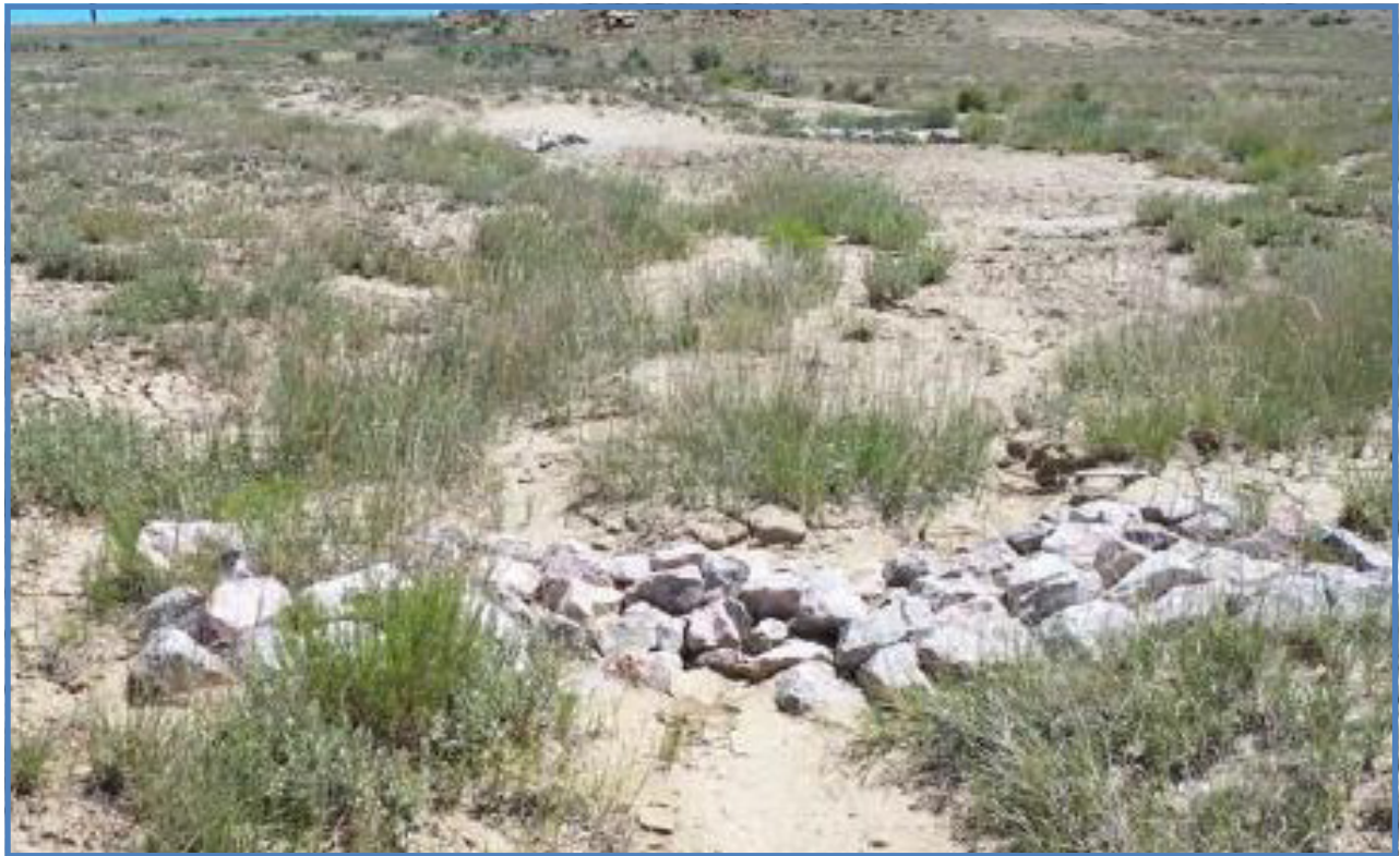
Photo above, example of a one-rock-dam. June 2023
