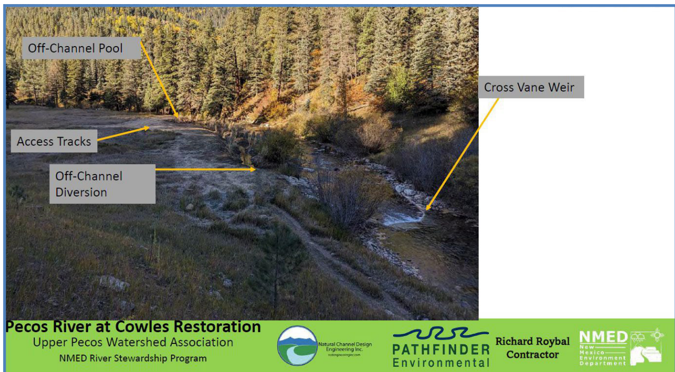
Photo above provided by Devin Kennemore of Pathfinder Environmental. This photo depicts the upper half of the project area looking downstream.
