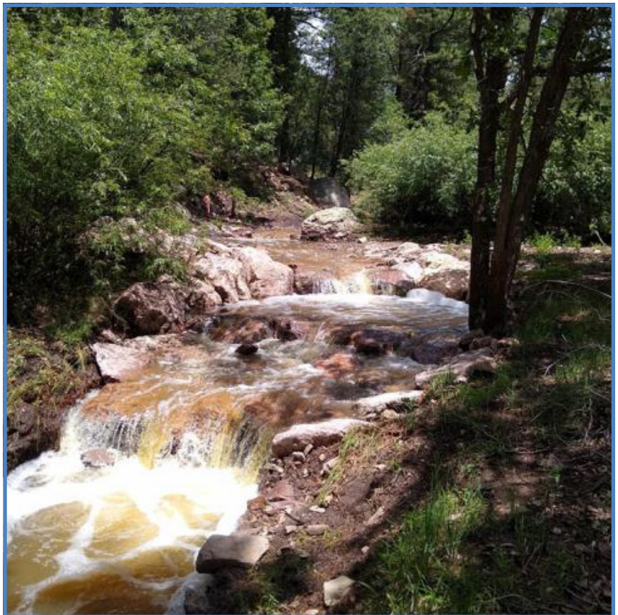
Photo above, Cherry Creek in flood, August 2022. The constructed Zuni bowls and step-down pools were built to address a 5-foot headcut in this location.
