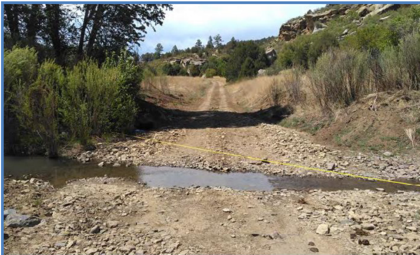
Photo above, Low water crossing 6 before treatment, June 2020.
