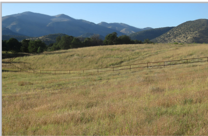
Figure 2. Mine waste was buried under a vegetated earthen cap at the Cowboy Flat Repository.
