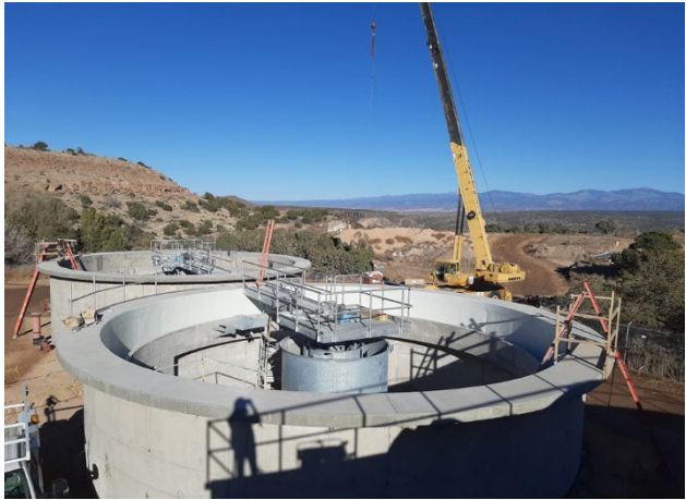
Los Alamos County CWSRF 083 Clarifier Construction.
