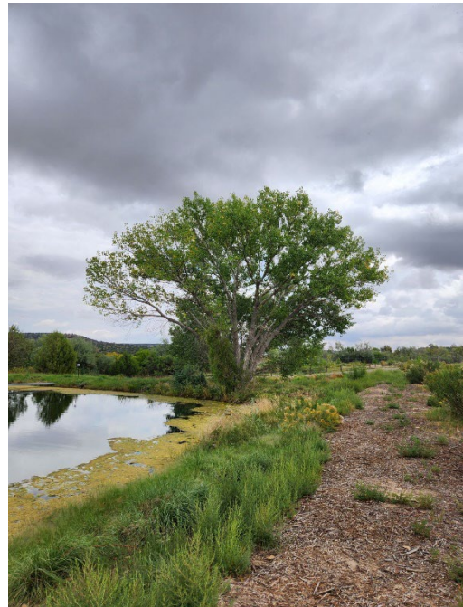
NMDGF Rock Lake Hatchery Settling Pond
