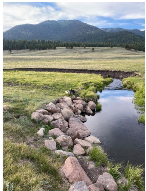
Rock armor to protect the road crossing at San Antonio creek above VC02 (stream temperature monitoring location)
