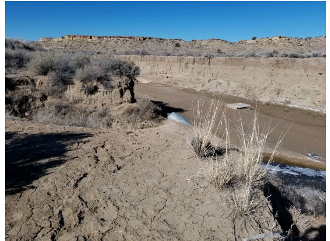
An outfall at the Gallup WWTP
