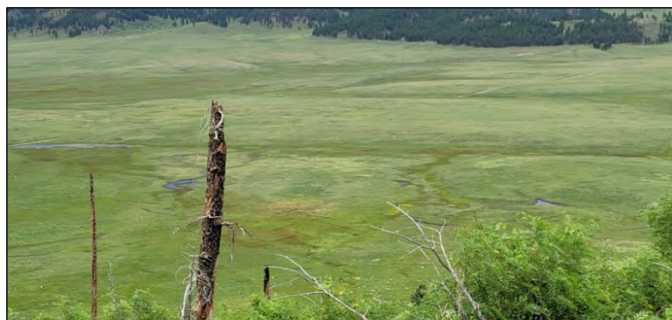
Plug and Pond Restoration Structures, East Fork Jemez River (photo Steve Vrooman)
