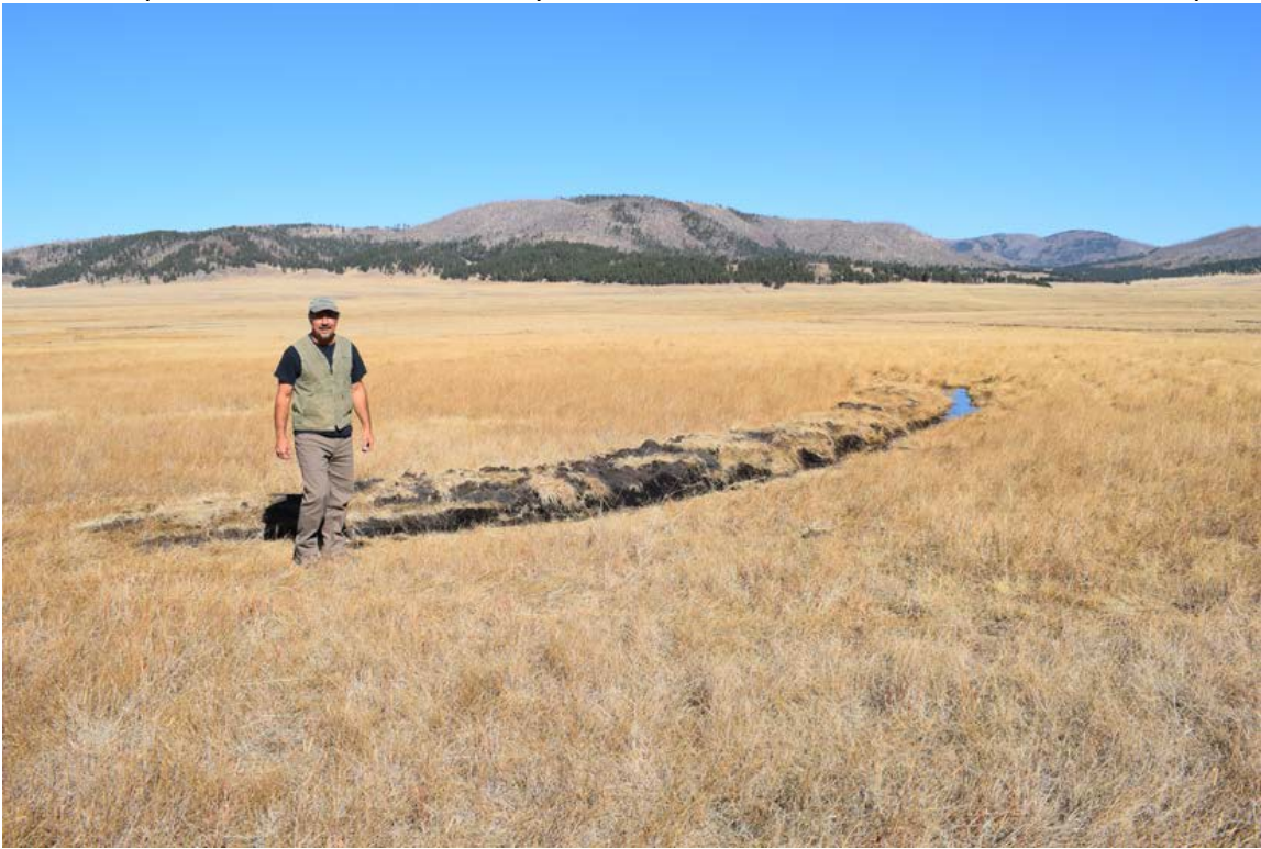
Figure 6 Subcontractor Steve Vrooman, Keystone Restoration Ecology, in front of a newly constructed contour swale that is partially filled with water.
