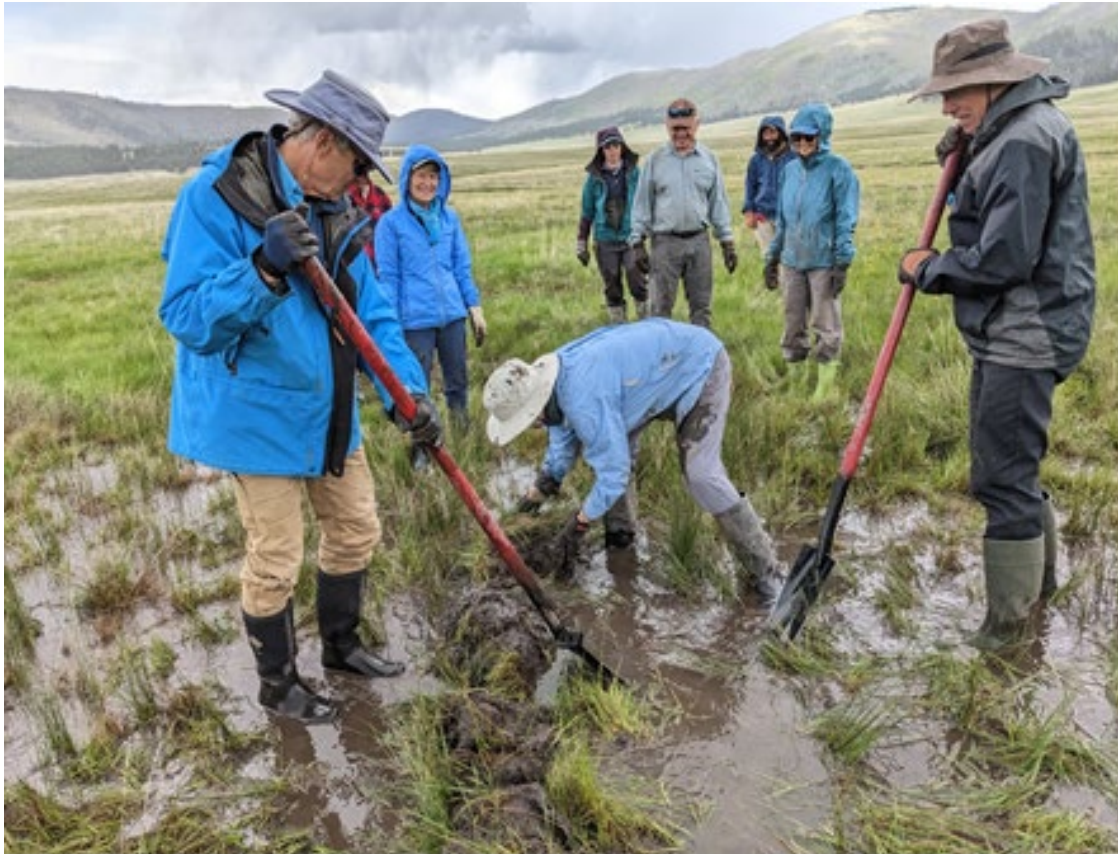
Figure 3 Volunteers for the Outdoors members building sod structures using wetland sod
