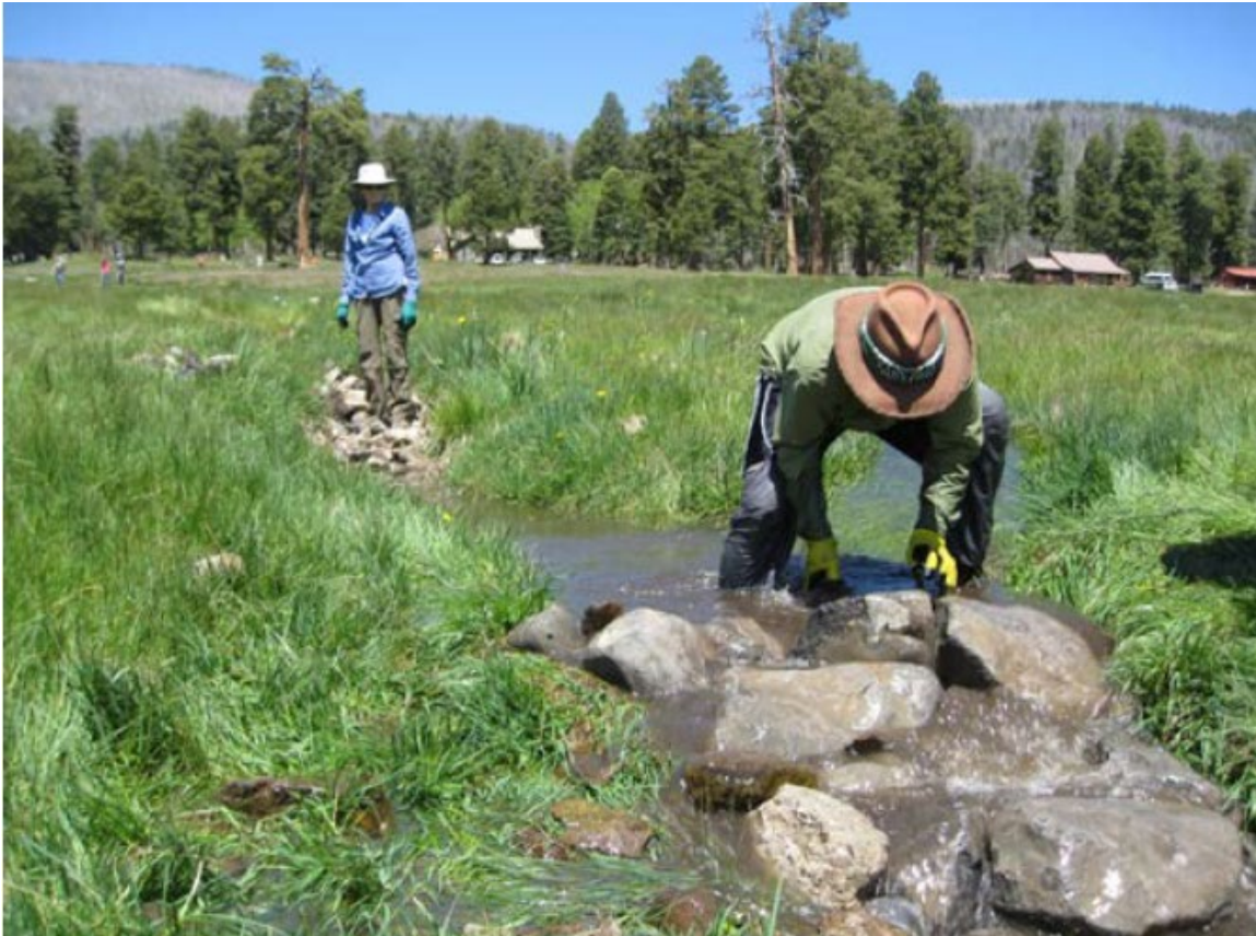
Figure 4 Albuquerque Wildlife Federation volunteers building a rock rundown structure that stabilizes the channel and spreads water into adjacent wetlands for the La Jara Creek project.
