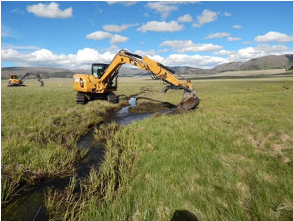
Figure 2 Subcontractor Keystone Restoration Ecology creating an excavator plug that will re-direct and spread water from the channel into historic wetlands.
