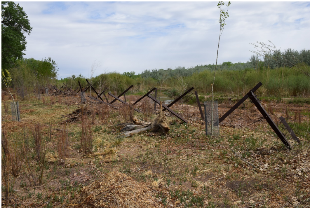
Figure 2-3. Photo of Jetty Jacks perpendicular to the Rio Grande.
