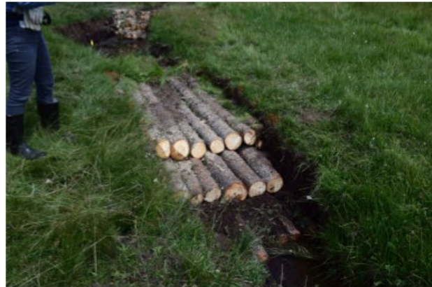
Log and Fabric Step Fall (K. Menetrey 2014)
