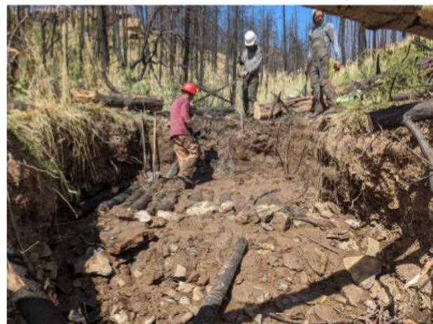
A crew constructs a Log Step Fall at a large headcut (P. Watson 2023)
