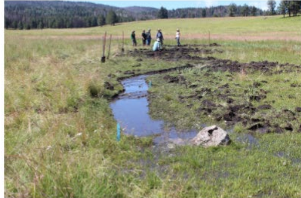
Hand-dug worm ditch (K. Menetrey 2015)
