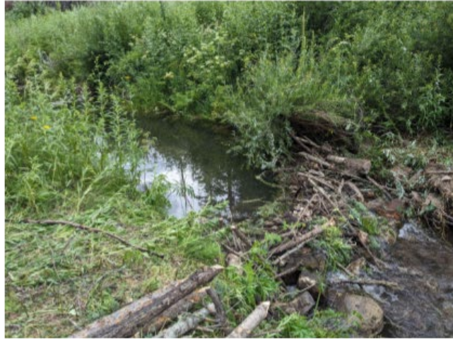
Postless BDA incorporating boulders and woody material (P. Watson 2023)
