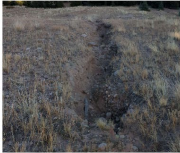
Gully caused by concentrated road drainage (P. Watson 2023)
