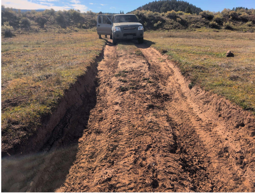
Figure 5. Road crossing the Camp Seven tributary showing significant incision and soil erosion. This road crossing connects Bluewater Creek to a long stretch of road on the terrace behind the truck that could be maintained to drain sediment into upland meadows instead of the creek.
