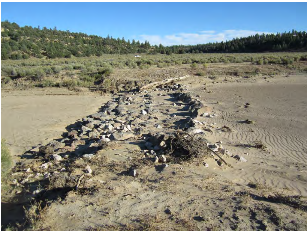
Filter Dam in October 2013, filled in with sand
