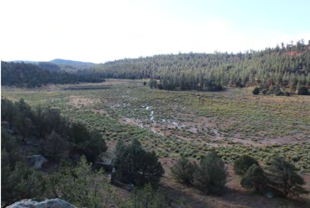
[Top left] Before plug and pond construction. [Top right] Water is once again accessing the stock tank benefitting the permittee. [Left] Water is returned to the Valley Bottom, increasing wetland potential.
