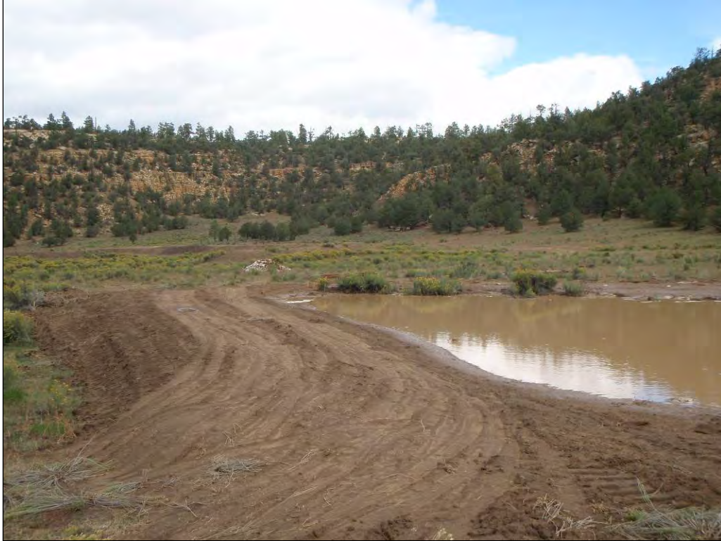
Detail of plug and pond at top of project, gully became a pond with overflow to left of picture. Pic October 2011.
