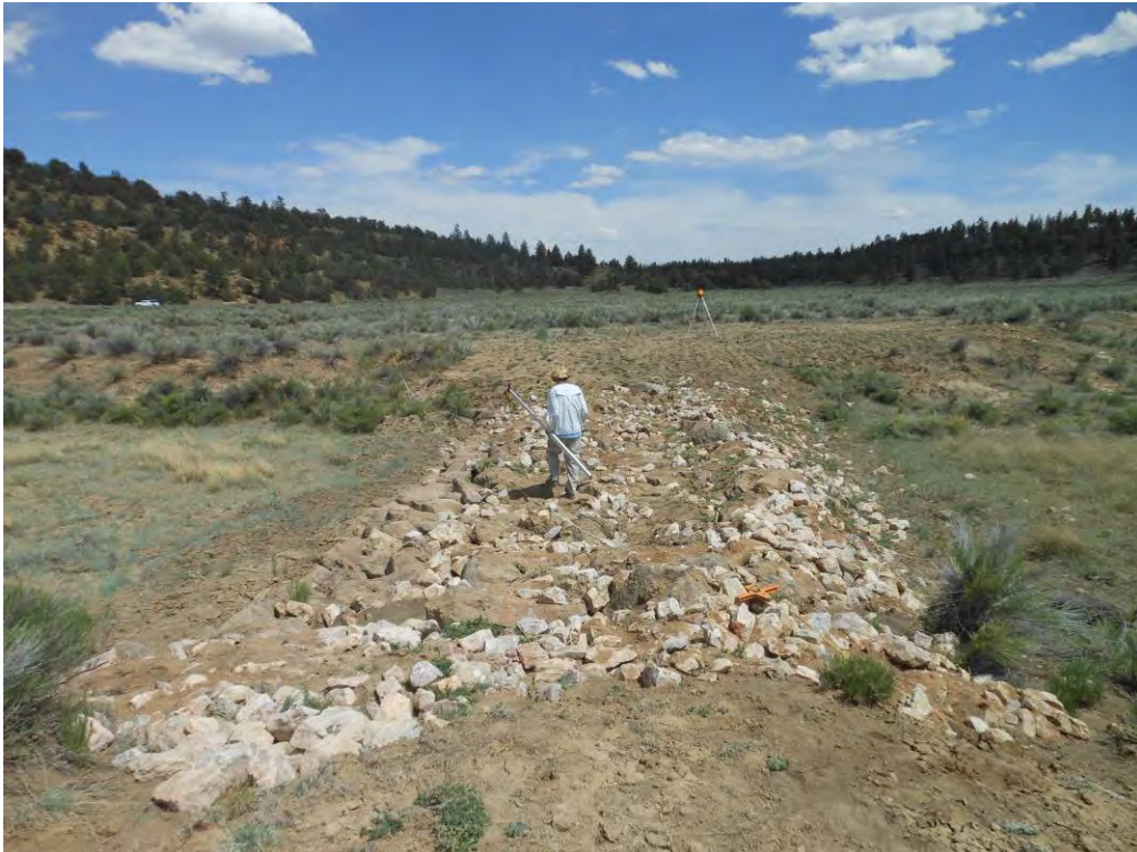
Filter Dam below Berm breach and channel reconstruction, spring 2012
