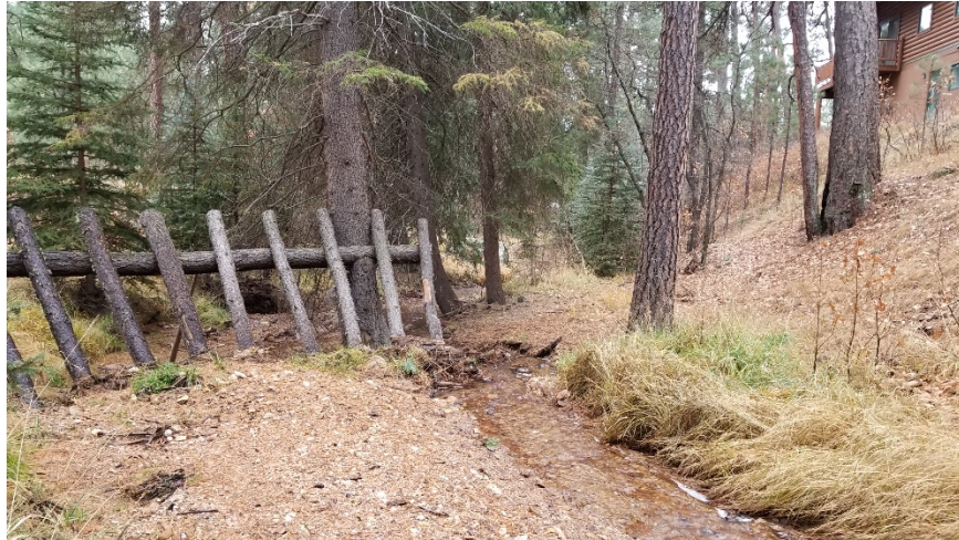
Figure 5-6. Trash rack built by the BAER Team to catch debris along lower Sulphur Creek after the Thompson Ridge Fire. Photo courtesy of Jim Counce.
