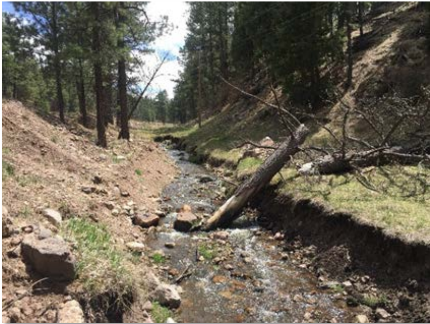
Figure 4-6. Scour along Redondo Creek that occurred from post-fire flooding after the Thompson Ridge fire. Photo courtesy of WildEarth Guardians.
