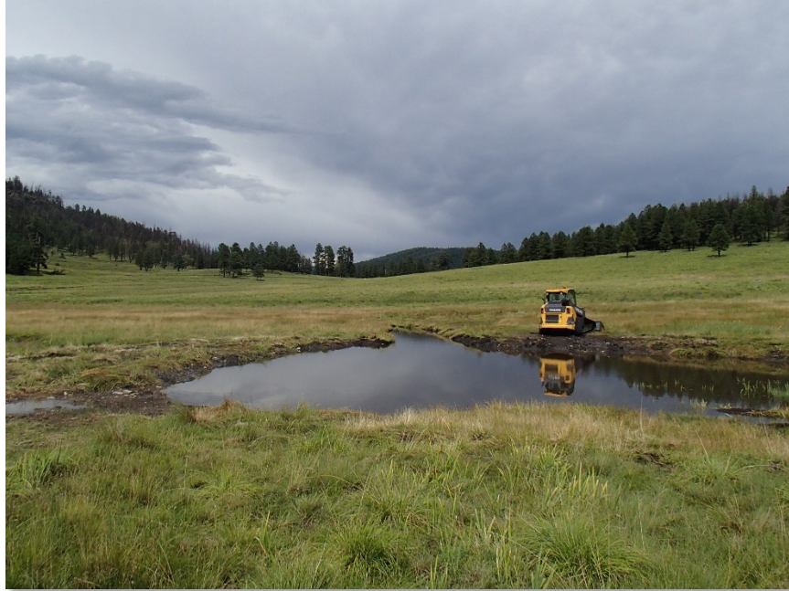
Figure 5-9. Plug and pond treatment in Valle Seco just after construction. Photo courtesy of Steve Vrooman, 2016.
