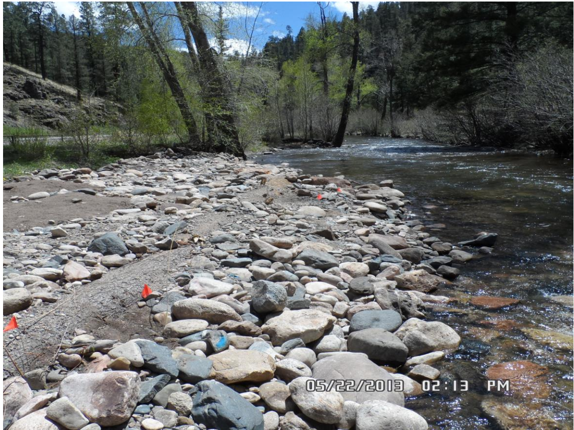
Figure 20. Streambank and riparian habitat improvement along the Pecos River near the Rio Mora confluence. Stream was narrowed, creating a wider planting zone for riparian vegetation.
