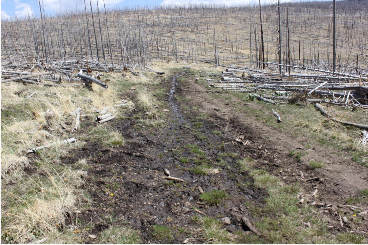
Figure 18. Slope type wetland at high elevation wetland with poorly sited road cutting bisecting the water flow.
