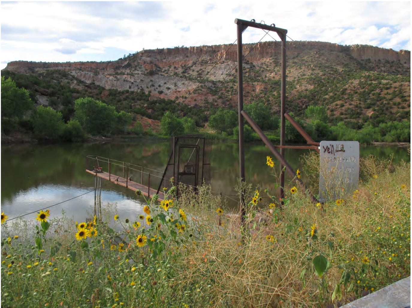
Figure 2.1 Pond and diversion structure above Ponderosa on Vallecito Creek. (Photo: SWQB staff, 8/30/2019)
