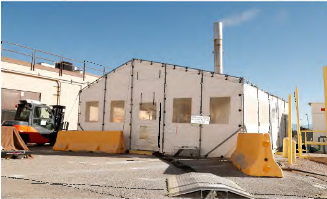
MES: Natural gas-fired mechanical evaporator
