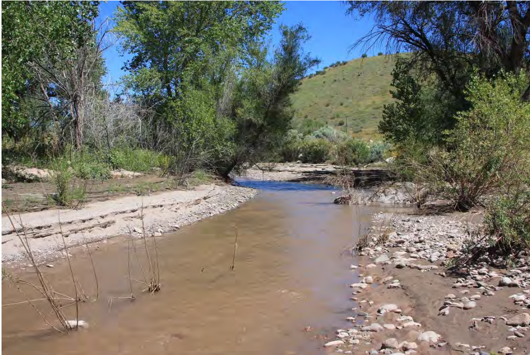
Fig A Royal John Bridge, Segment 20.6.4.803 (upstream view)
