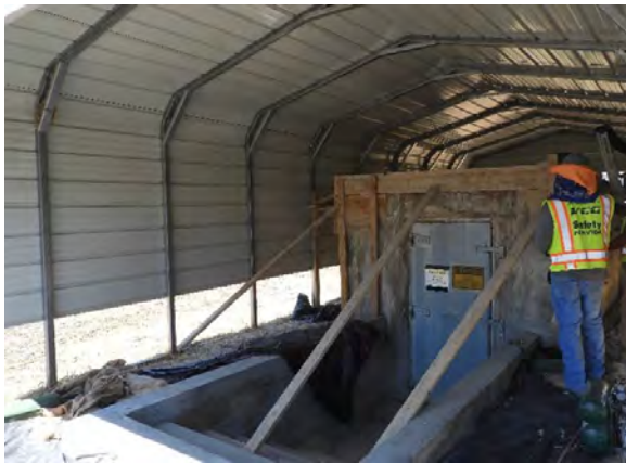
Figure 3-2. Bunker 18-2 during concrete restoration in July 2019
