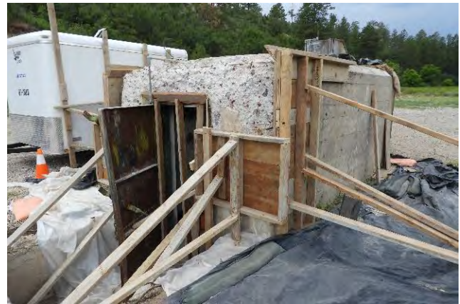
Figure 3-3. Bunker 18-5 during concrete restoration in July 2019
