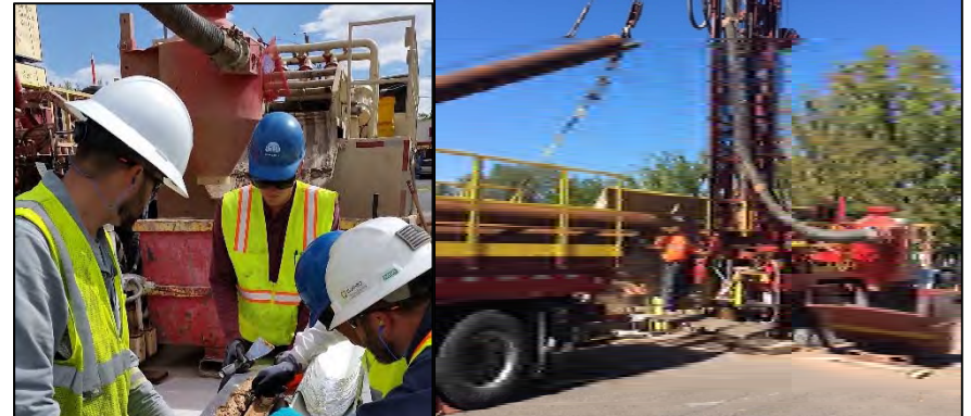
Well installation in neighborhoods
