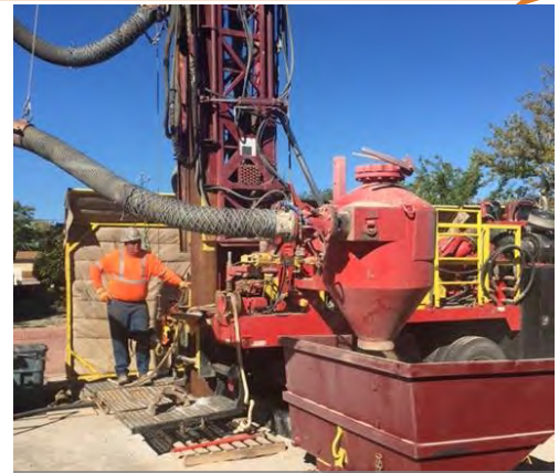
Using ARCH drill groundwater monitoring well
