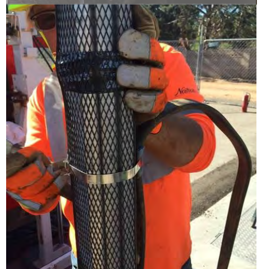
Installation of anode on extraction well pump for corrosion protection (Summer 2016)
