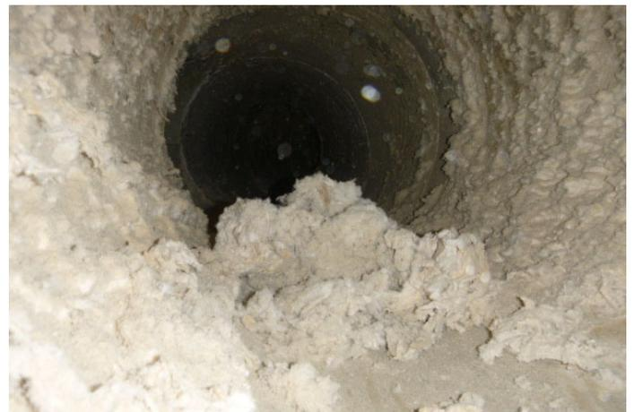
*If air velocity in baghouse intakes falls below the minimum require to keep dust in suspension it will settle out and restrict air flow even more.*
