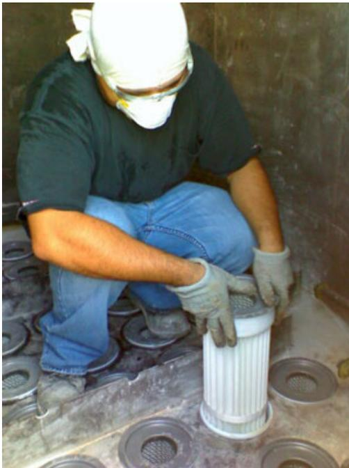
*Filter media should be inspected and replaced regularly to keep a baghouse operating at high efficiency.*
