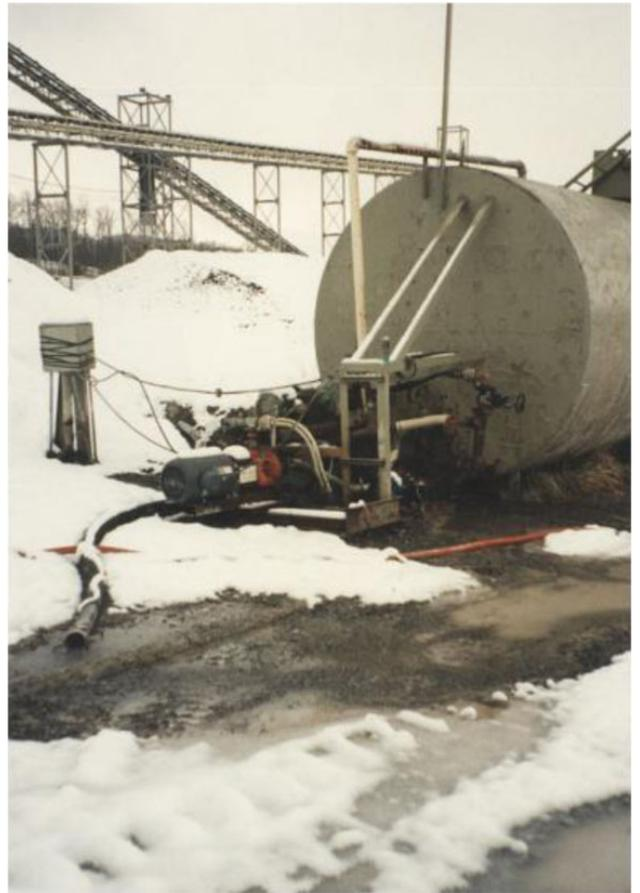
*Spray system pumps and components should be housed in heated enclosures to protect them freezing.*
