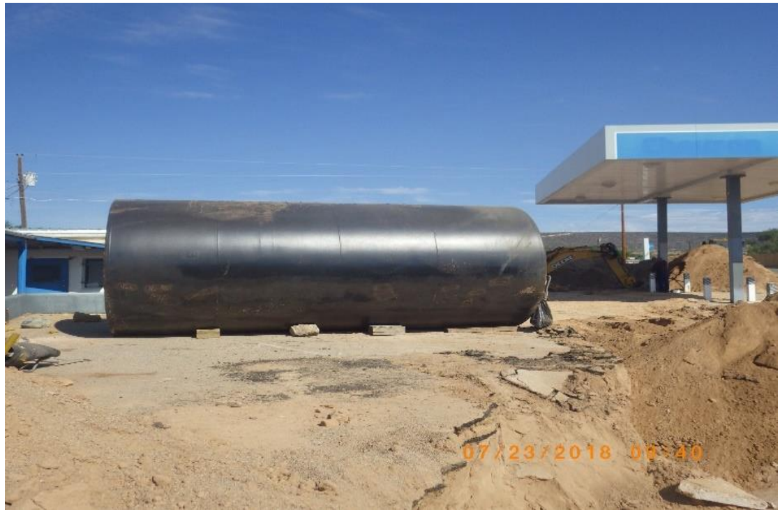
Photo: Tank Removal at Ohkay Owingeh Overseen by PSTB
