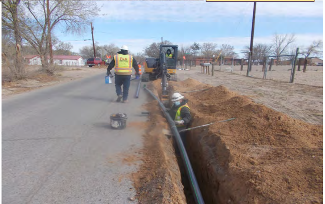
Construction of low pressure sewer collection line
