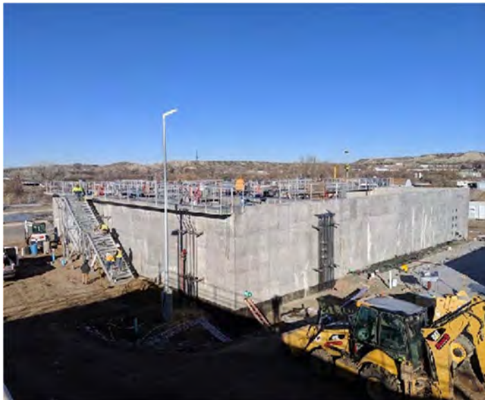
Sequencing Batch Reactor Digester
