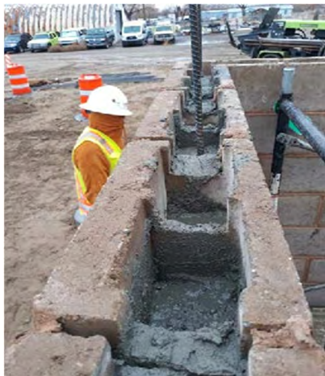
Grouting block cells and bond beam at Chemical Building CMU –City of Bloomfield
