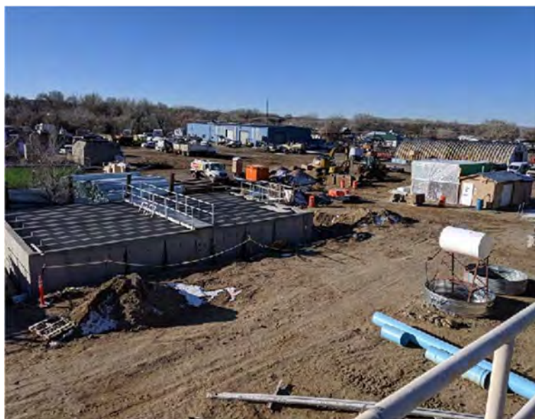
City of Bloomfield-Chlorine Contact Chamber
