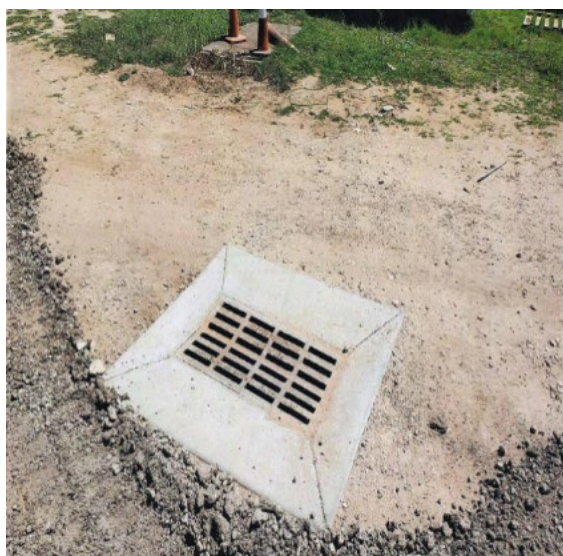
Flooding at Roosevelt County Fairgrounds (above) and storm water inlet constructed to address the problem (below)
