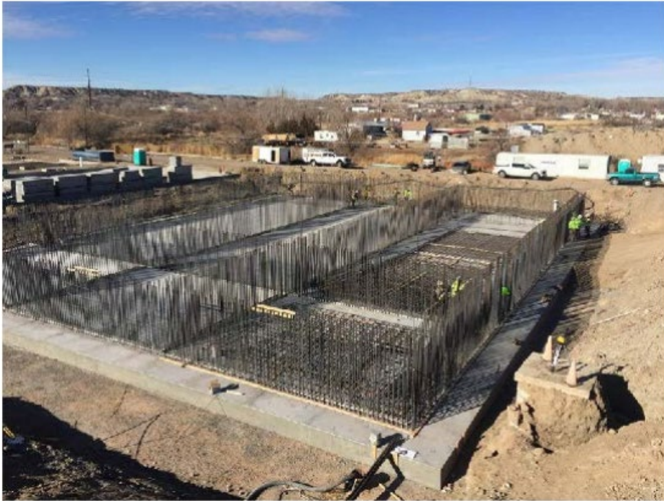
The Town of Bloomfield CWSRF 103 WWTP Construction
