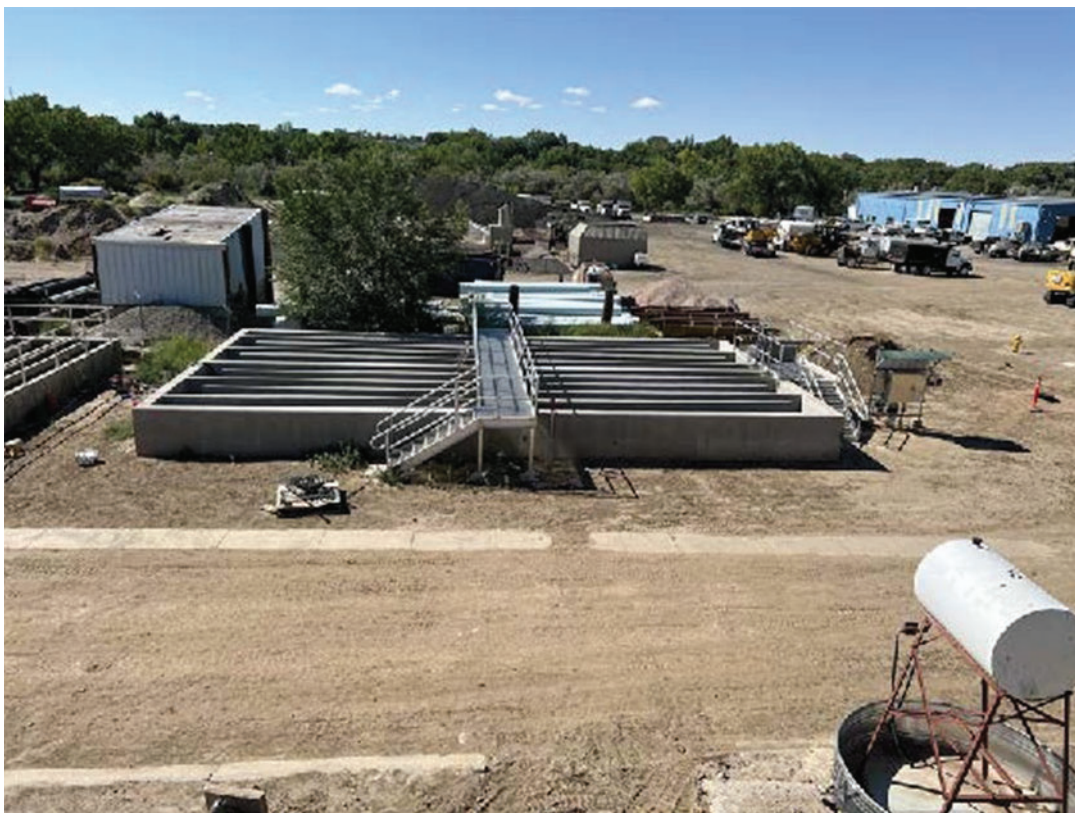
Bloomfield CWSRF 103 Chlorine Contact Chamber
