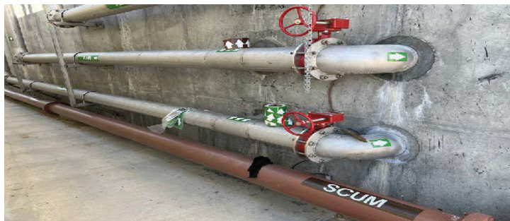
Bloomfield CWSRF 103 Pipes with Directional Arrows
