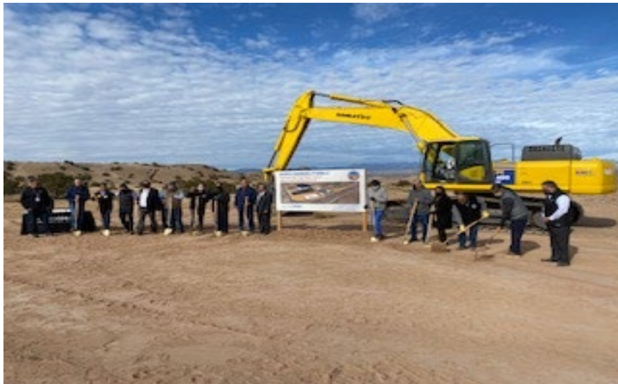
NMED in attendance and support of the first shovels of dirt moved in preparation for Kewa Pueblo’s Wastewater Treatment Plan Groundbreaking Event on December 8, 2021
