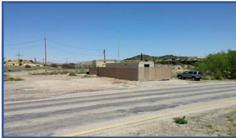
Pictured is a soil vapor extraction system at the Laguna Mart release site
