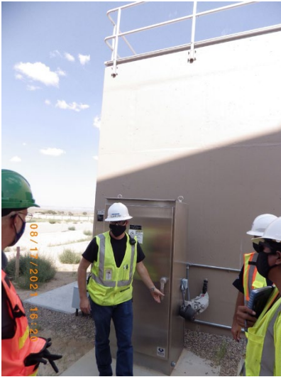
Cutter Lateral Treatment Plant Sanitary Survey
