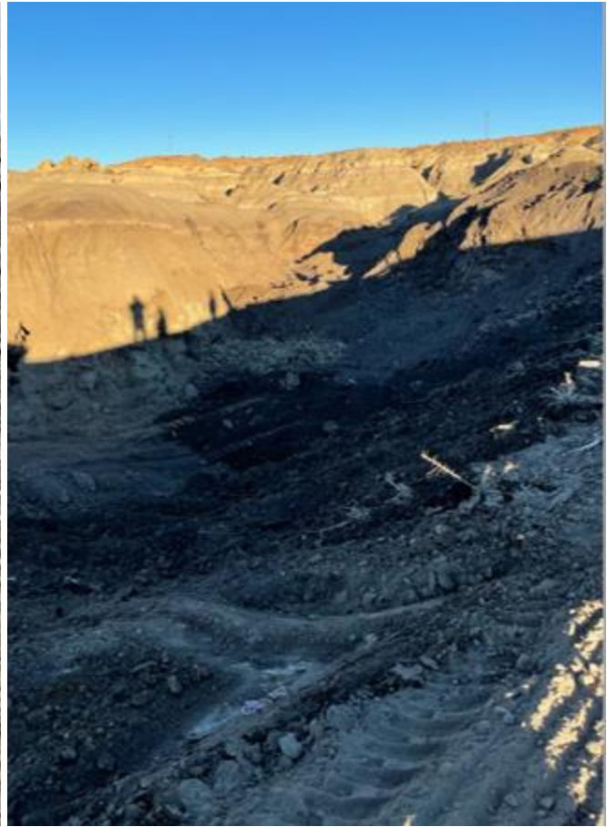
Site after abatement was completed
