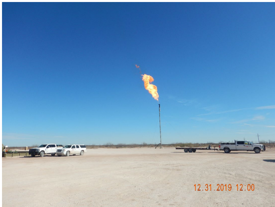
An unauthorized flare at Ameredev's Nandina facility, photo by AQB inspectors taken on Dec. 31, 2019.
