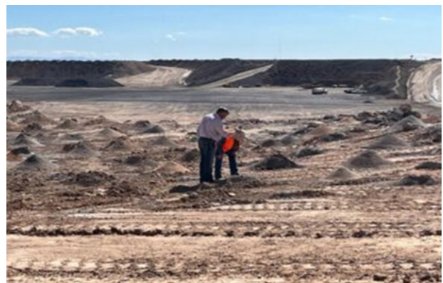
Eric Gordon learns how new areas are blasted at the Los Lunas quarry.
